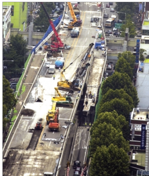
Demolition of Samilro elevated road
