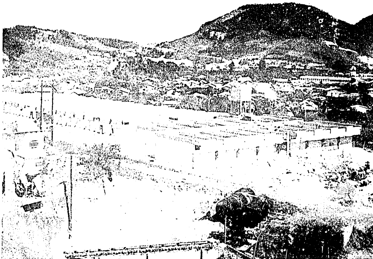
Figure 6 TECHNOLOGY CENTER UNDER CONSTRUCTION FESSC, JANUARY 1978
