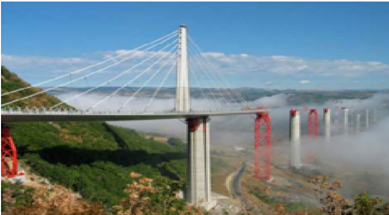
Photo 10: Launch L4S after re-tensioning of the stay cables
