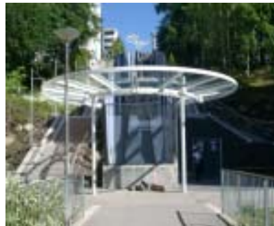
{Figure 11} Vertical Passenger Lift (Stockholm, Sweden)
