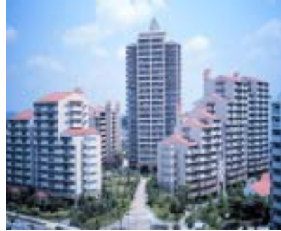
{Figure 9} Various Building Heights (Kobe, Japan)
