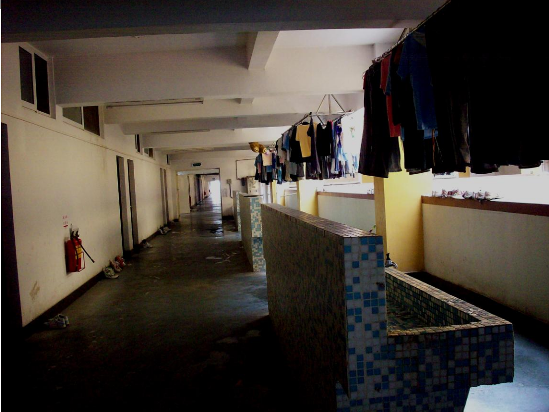
Images: Dormitory hallway
