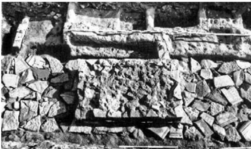
213 Rome, SS. Marcellino e Pietro. Foundation built with grave stelae of the equites singulares .
