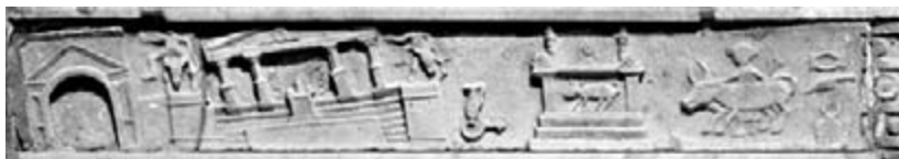
207 Relief depicting an earthquake, H. 16.5 cm. Pompeii, House of L. Caecilius Iucundus.
