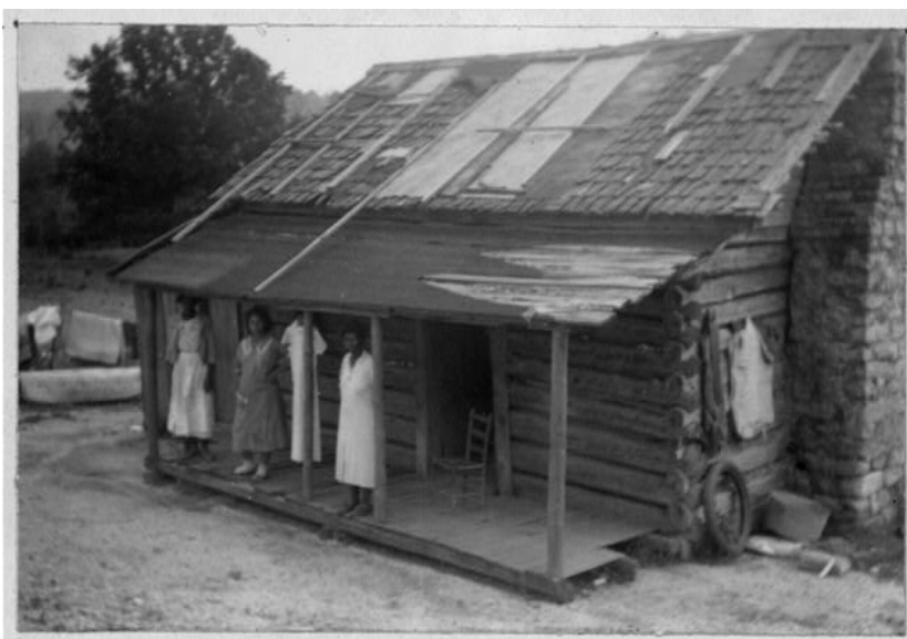
Ilustración 8 Abraham Jones' House. Alabama United States, 1936. Between 1936 and 1938. Fuente: Photograph. https://www.loc.gov/item/mesnp010233c/ .
