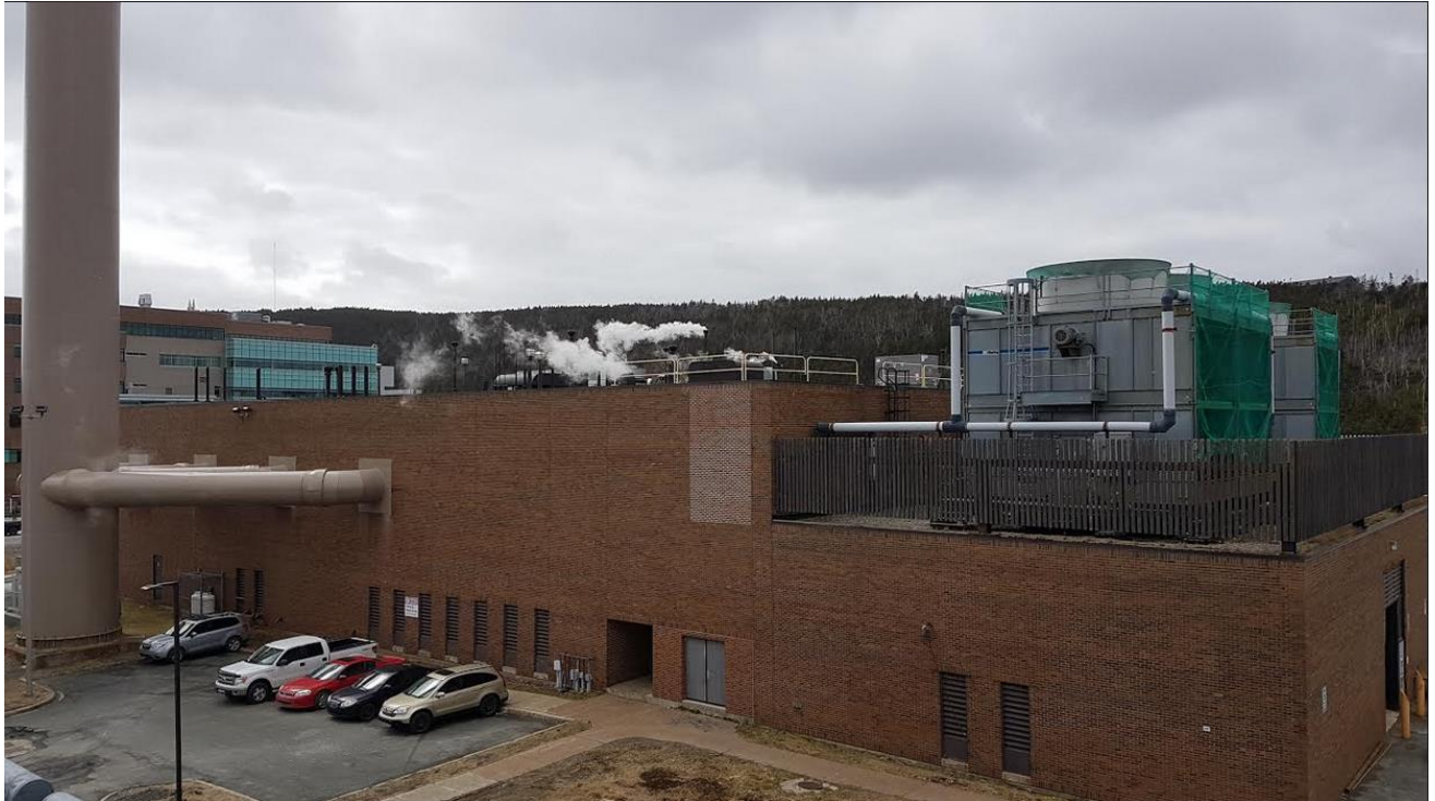
Figure 1.2 The main campus heating plant
