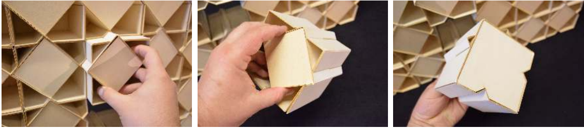
Figure 7.10 – Grip and pull. The design of the blocks allows the easy gripping and pulling of blocks out of the wall. Image credits: the author.
