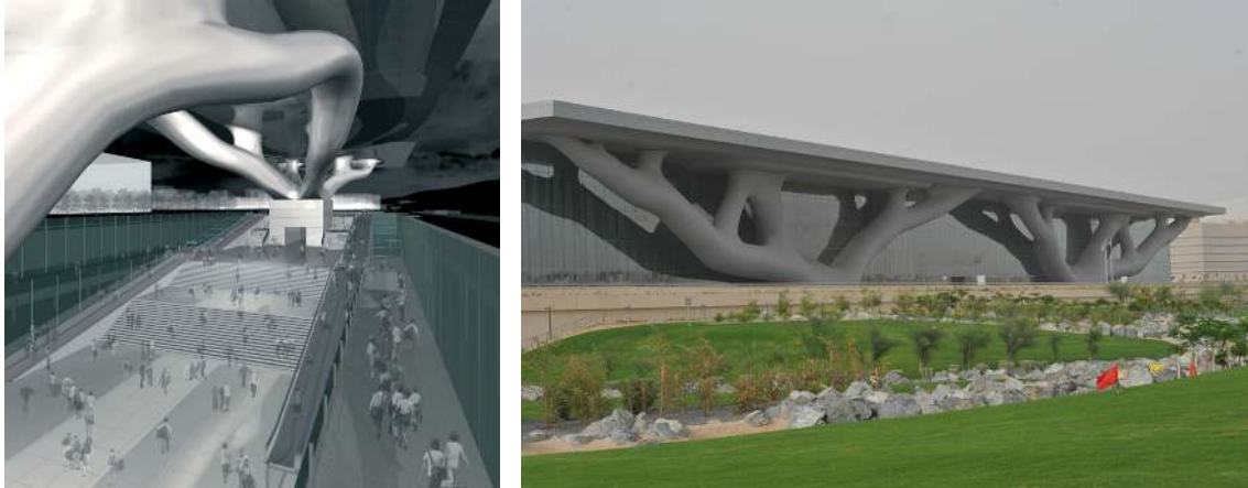
Figure 3.35 – Topology optimization. Architectural design using topology optimization as generative design technique in the work of Arata Isozaki with engineer Matsuho Sasaki. Left: Florence Train station competition entry. Right: Qatar Education City Convention Center. Image credits: Sasaki, Itō and Isozaki 2007; Dapogny et al. 2017.
