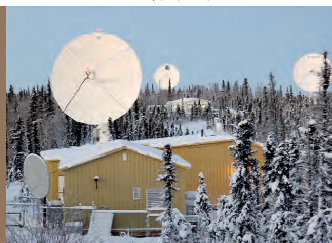
International Satellite Station Facility (ISSF) Inuvik, Kanada
