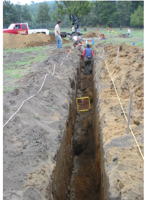
Figure 32. Overview of South Trench, facing north.
