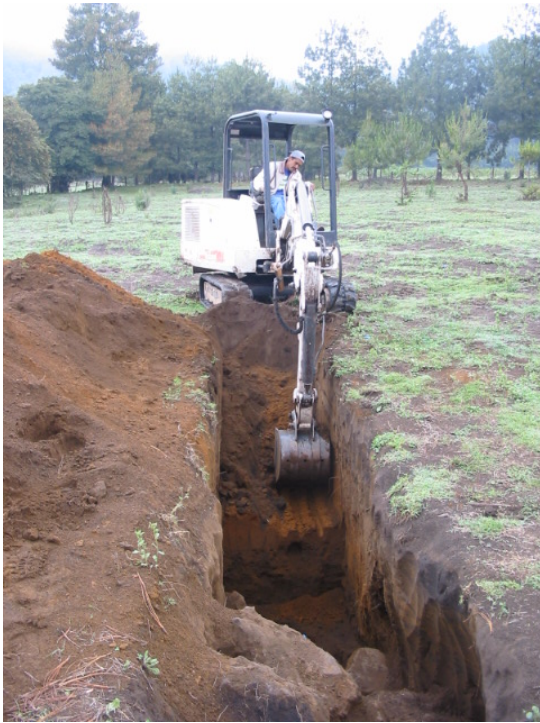
Figure 29. Photo of backhoe excavations.
