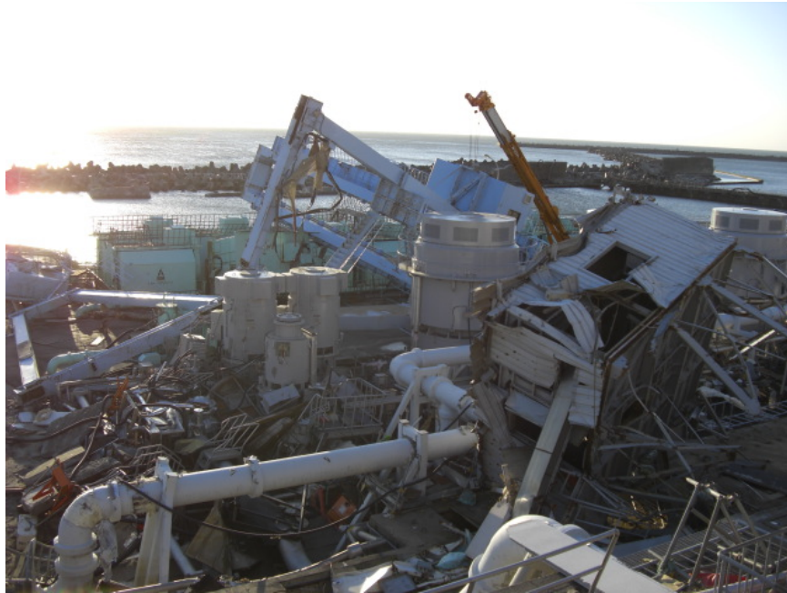
Fig. 5: Damage to the Fukushima Daiichi nuclear plant and indication of its proximity to the sea. (Source: Tokyo Electric Power Company 2011. Reproduced with permission)
