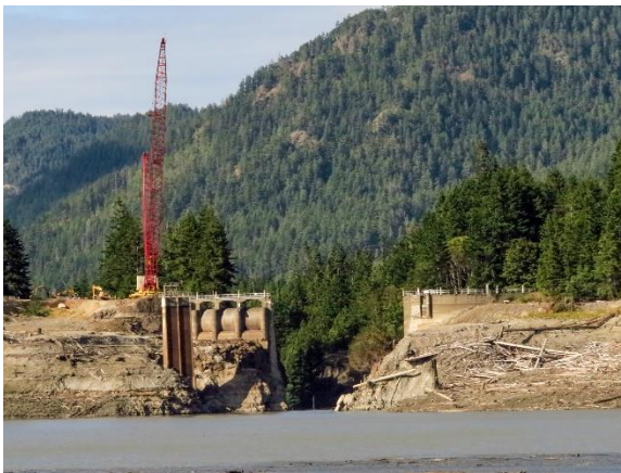
Figure 2: Glines Canyon Dam from the Lake Mills Reservoir taken August, 2012 prior to the coarse sediment release. Dam removal had already begun in June 2011 however, only suspended sediment was flowing at this point. (Photo taken by Bryon Free)
