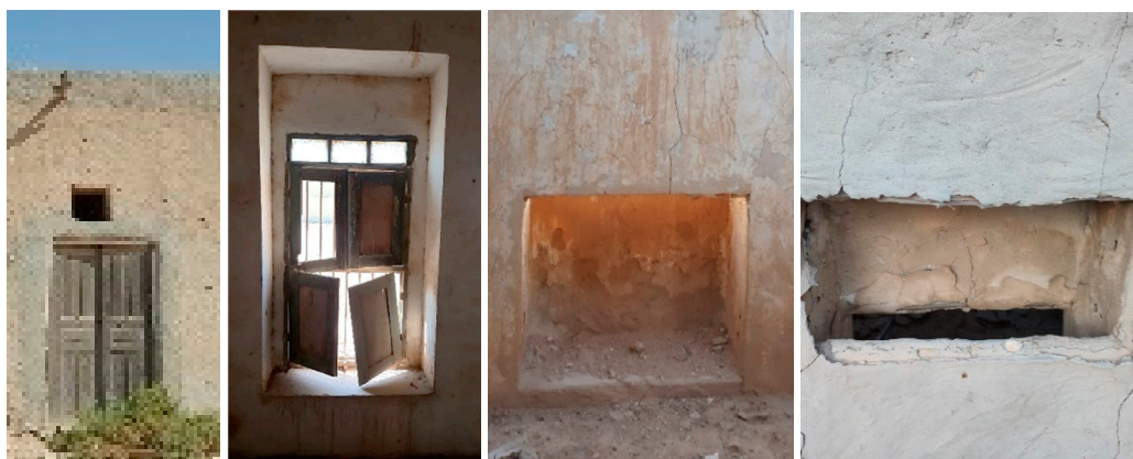
Figure 17. From left to right, Picture 1 shows a permanent opening above the room entry door used for cross ventilation. Picture 2 shows the details of the window. It has four shutters to reduce the daylight and to provide privacy. In addition, there is a row of three fixed glass panels on the top. Its location above the visual level ensures privacy to the occupants. Pictures 3 and 4 show the malqaf, the first from inside the room and the second from outside.
