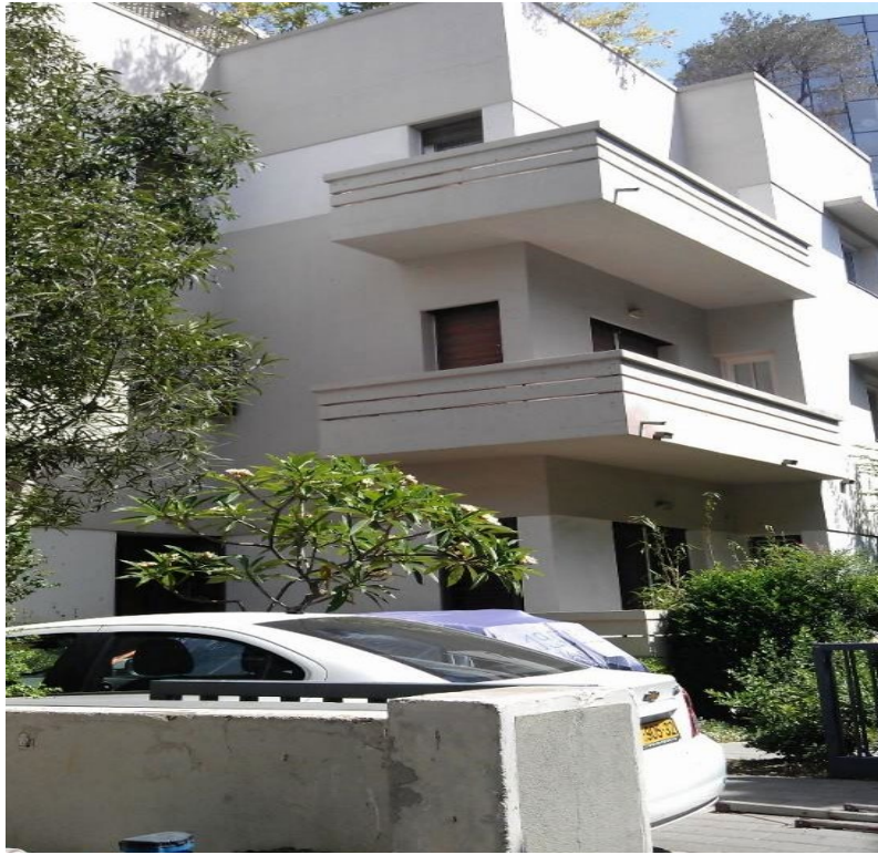
Figure 38: A Bauhaus building on Rothschild Blvd. 2018. Taken by the author.
