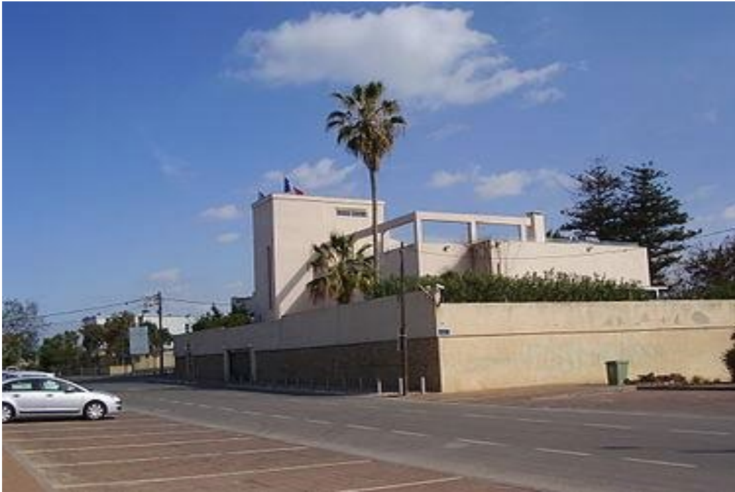
Figure 25: The French Ambassador's house in Jaffa. The North-East angle of the house. (see link above).
