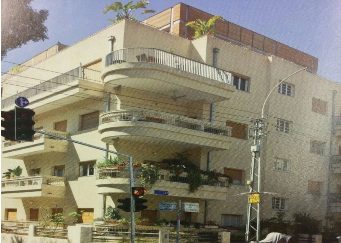
Figure 37: A Bauhaus building on the corner of Rothschild Blvd. and Balfour St. 2018. Taken by the author. In this picture one can see that another floor was added on top of the building, yet it is built further inside, not disturbing the sight of the façade of the original Bauhaus construction.
