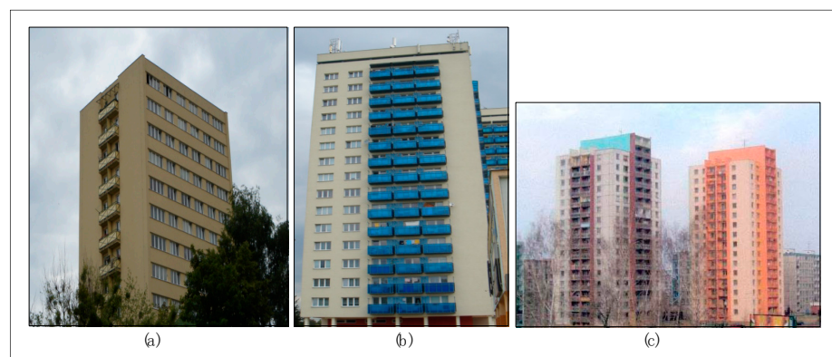
Figure A3. Prefabricated residential housing buildings after the renovation intervention by ETICS: (a) VOS system; (b) VMOS system; (c) VPOS system.
