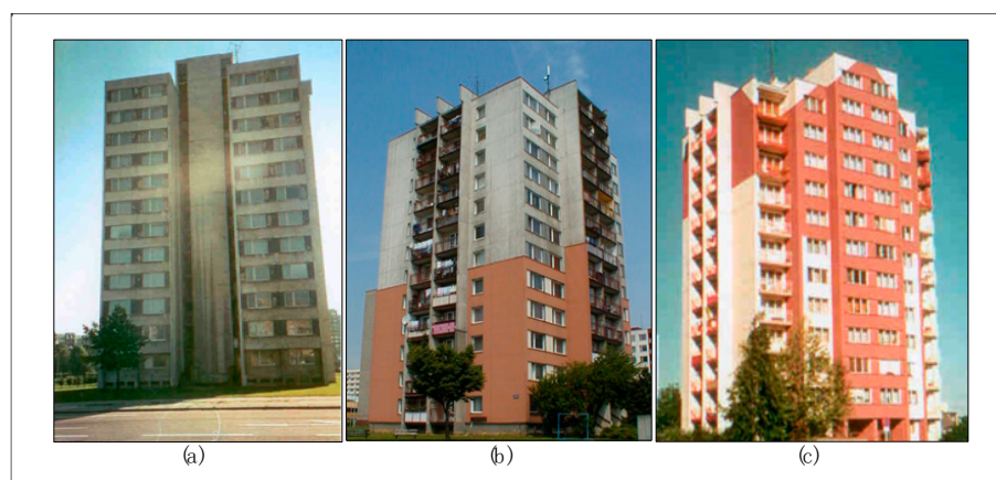
Figure A4. Development trends in the application of additional contact thermal insulation shown with an example of a prefabricated panel system of a residential housing building in the type series T06B-OS: (a) Prefab building in its original state; (b) lamellar contact design; (c) prefabricated residential housing building after application of ETICS.
