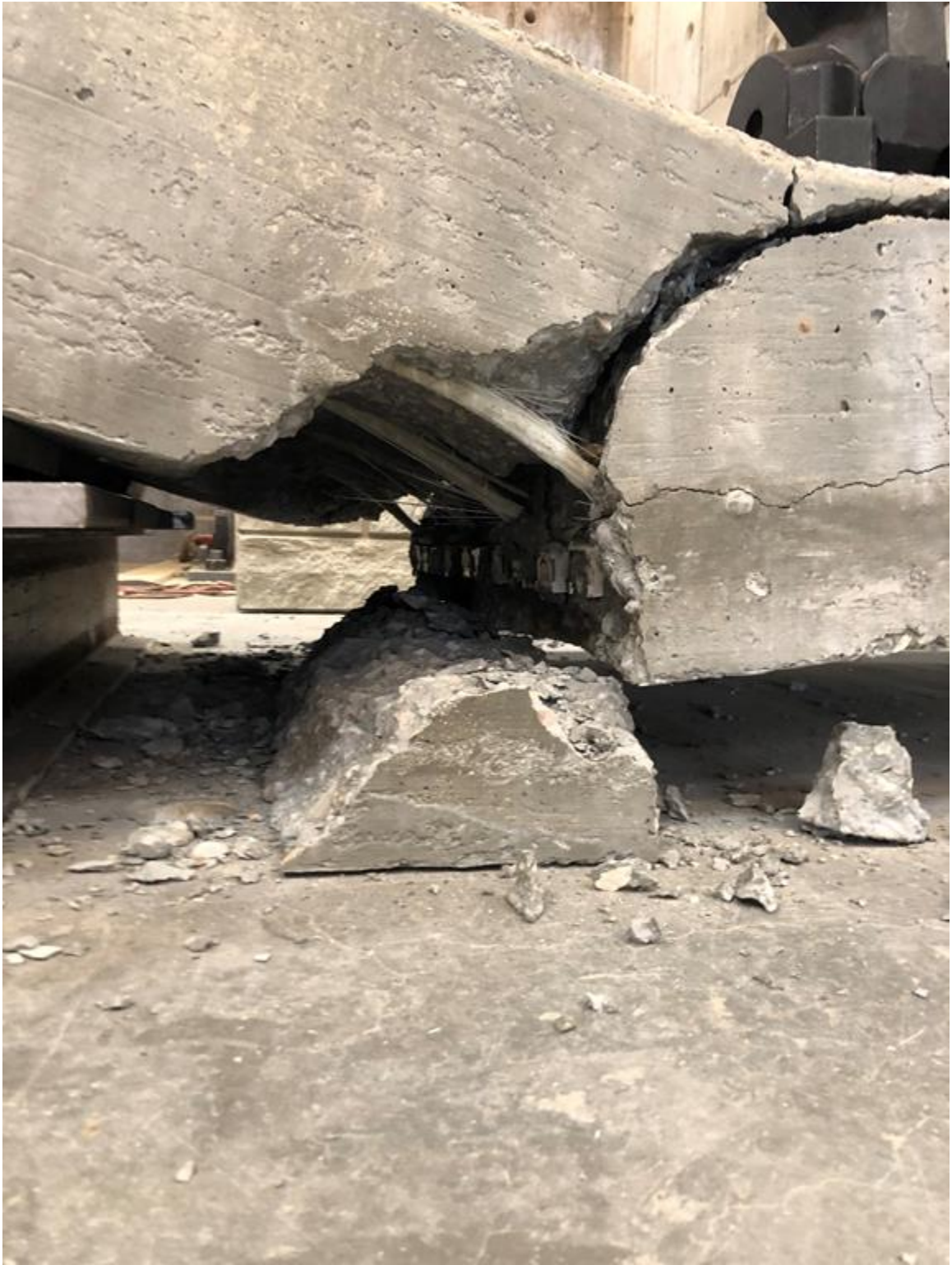
Figure 5-22 GFRP Reinforcement Failure
