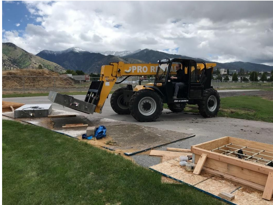
Figure 3-3 Moving the Slabs
