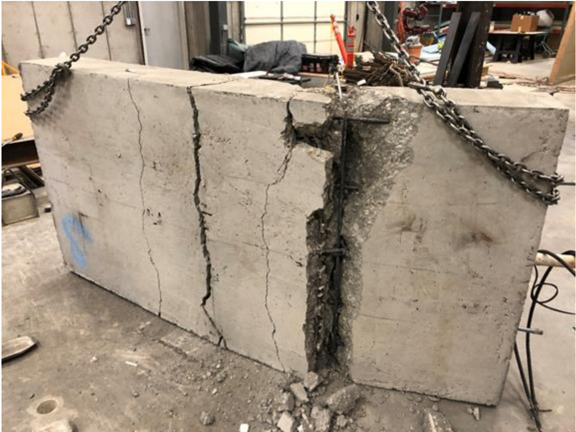
Figure 5-13 Face of Steel Reinforced Slab After Failure
