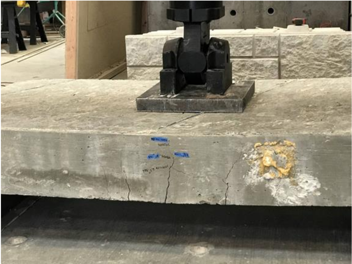
Figure 5-20 Cracking During Static Test
