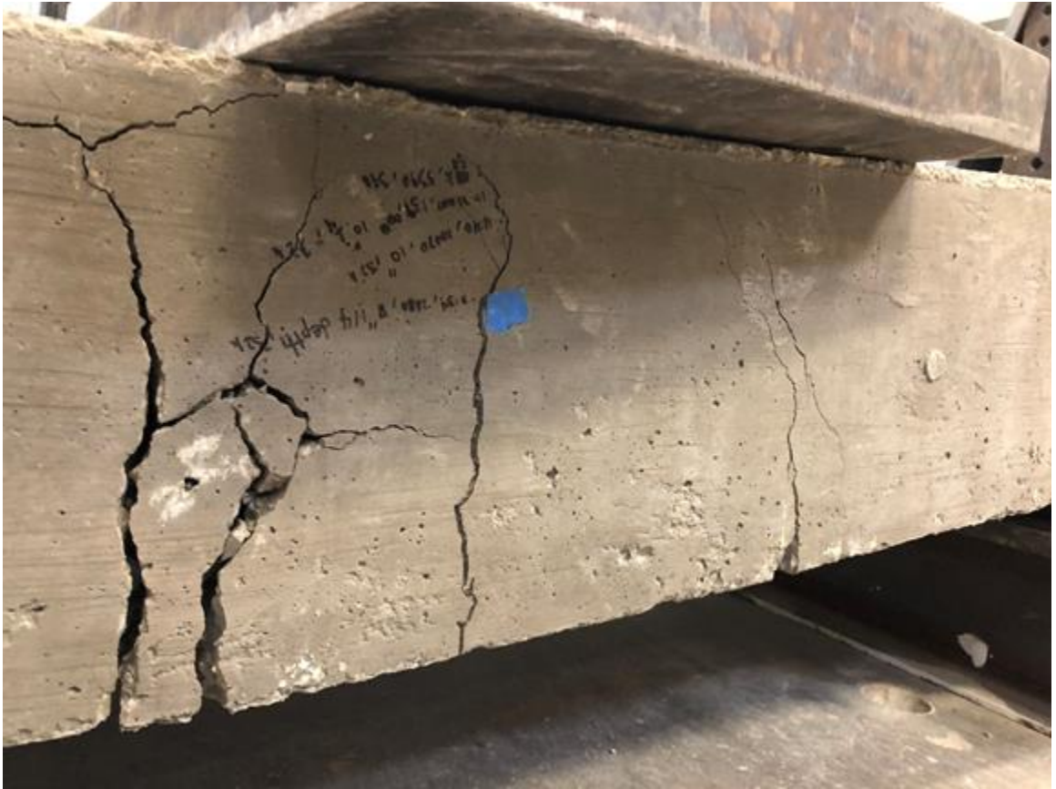
Figure 5-7 Steel Cracks Reverse Side
