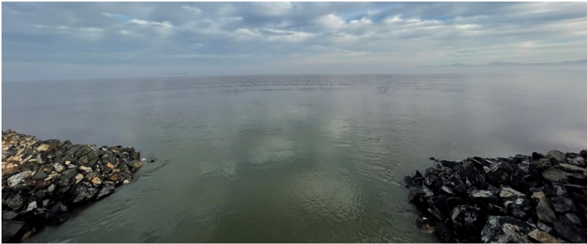
Figure 5.11. View from the WC breach at the Great Salt Lake Causeway looking north. Surface flows move from south to north (bottom to top of photo). Note the radial pattern at the surface, providing indication of the relatively lighter water from the south floating over the heavier northern water. Similar radial mixing pattern at the surface can also be observed in the CFD simulation (see fig. 12).
