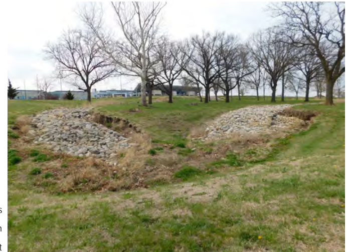
Figure 1.9. Bioswales and trees that take on drainage from the East Stadium parking lot
