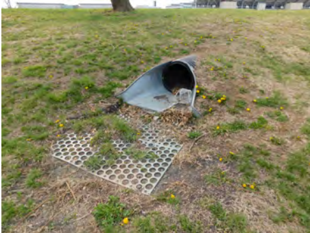
Figure 4.14. East Stadium parking lot storm sewer outlet.
