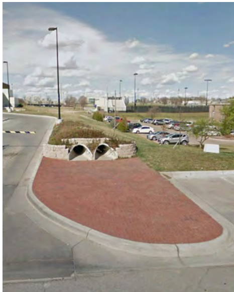
Figure 4.29. South Recreation Parking Lot southeastern stormwater outlet.
