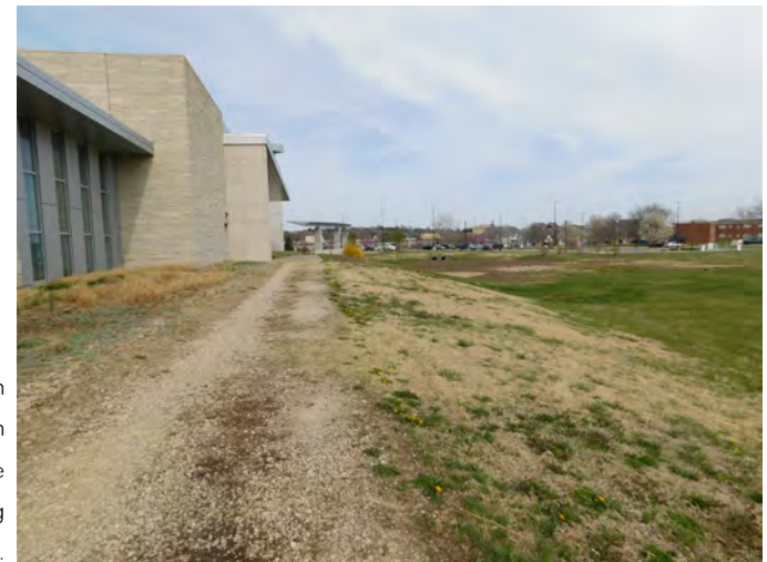
Figure 1.10. Detention basin south of the Peter's Recreation Center that takes on drainage from the East Stadium parking lot.
