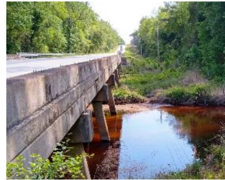
Bridge Scour Assessment and Management System, SCDOT
