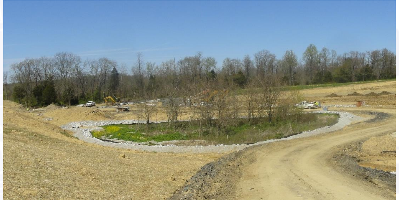
Rock ring U.S. 50 North Vernon Bypass
