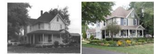
The James H. Chaddock Residence, 742 North Main Street This two story Queen Anne style design has a Colonial Revival style
