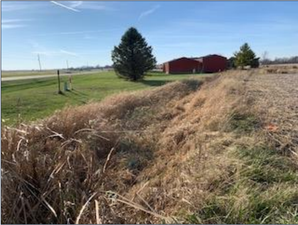
Dry Grass Swale, Hendricks County, Indiana
