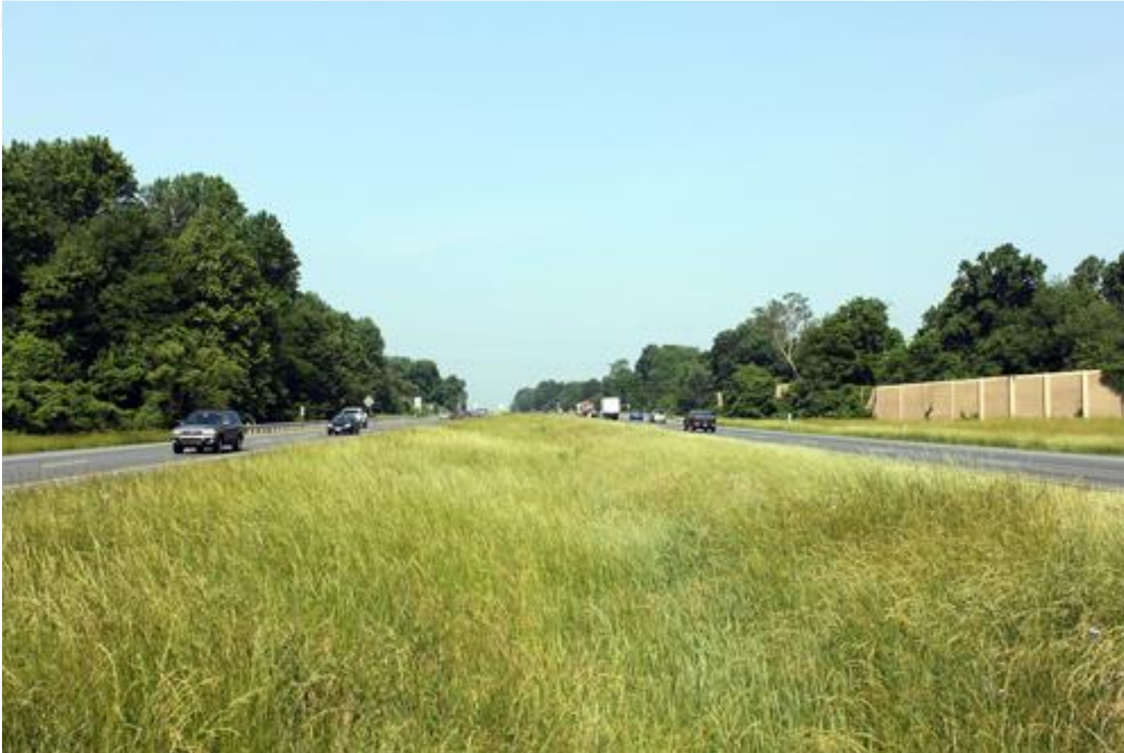
Grass Swale in I-70 Median – Maryland DOT State Highway Administration
