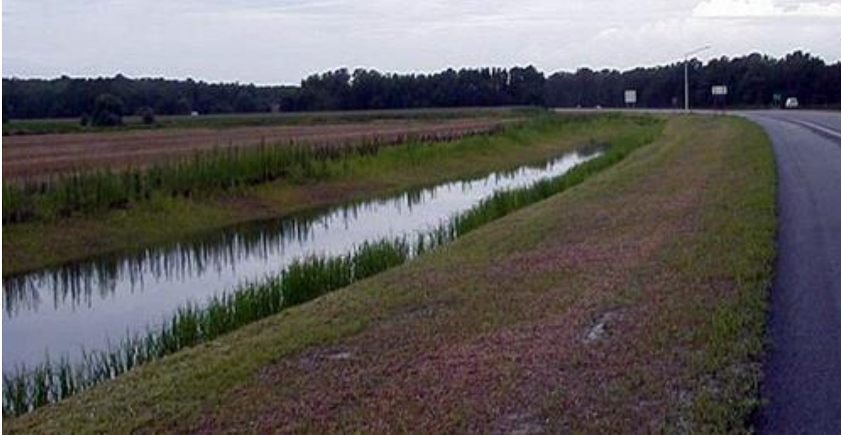
Wet Swale along US 113 – Maryland DOT State Highway Administration
