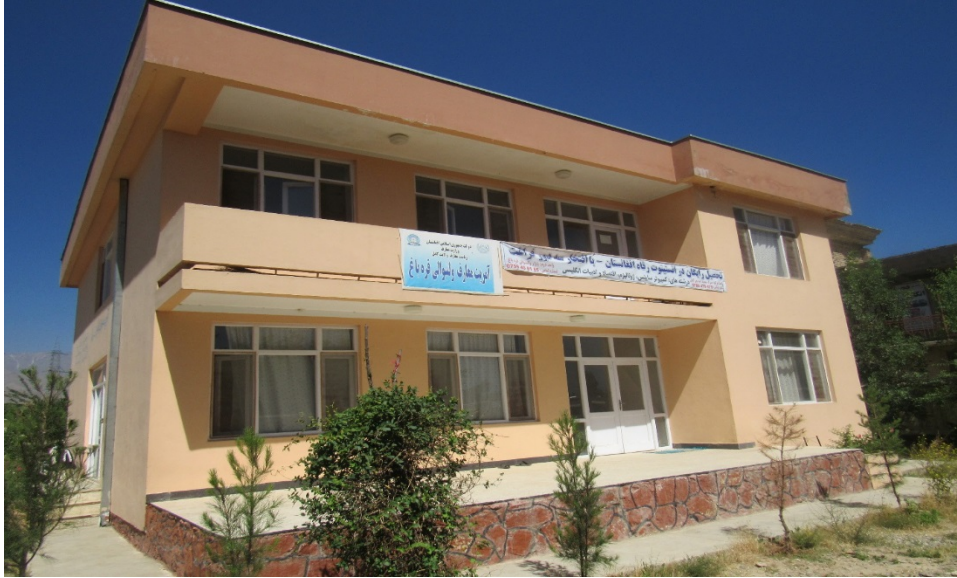
Figure A-31. Kabul School Admin 16 (front view)
