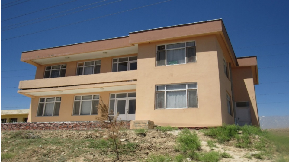
Figure A-33. Kabul School Admin 17 (front view)
