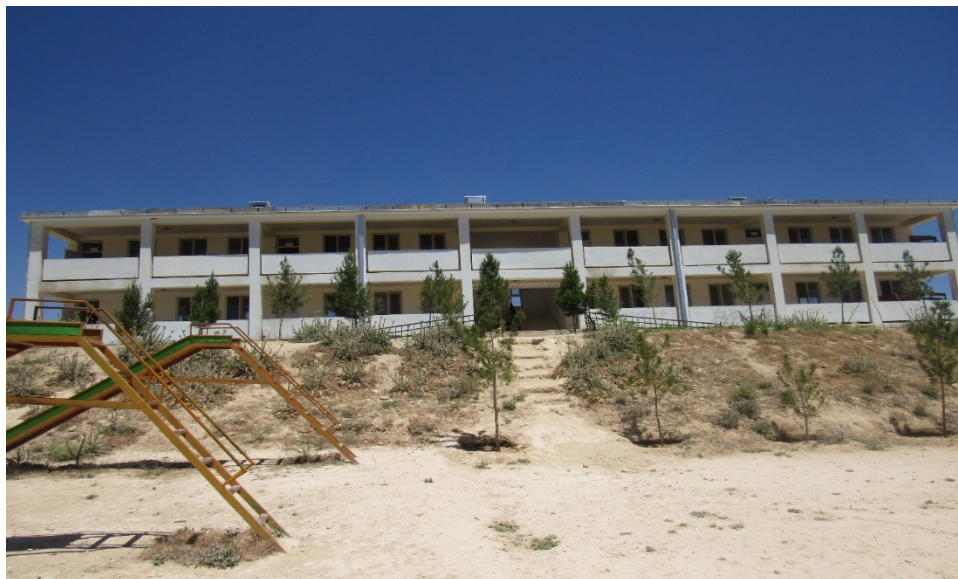
Figure A-55. Kabul School 28 (front view)
