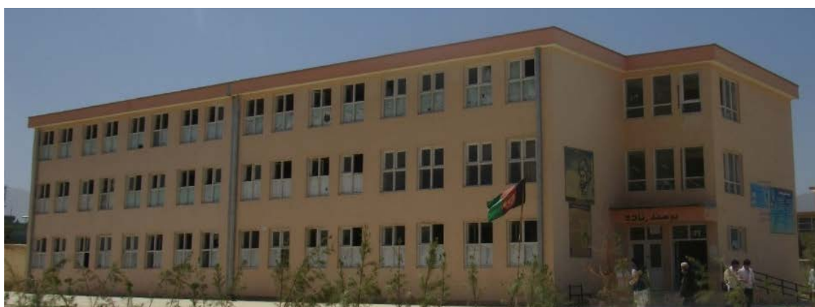
Figure C-2. Kabul School 49 (Front View)
