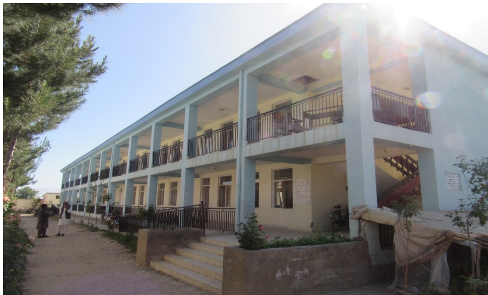
Figure A-53. Kabul School 27 (front view)
