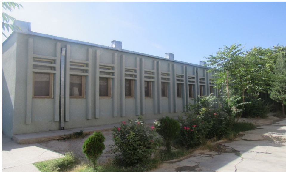
Figure A-39. Kabul School 20 (front view)
