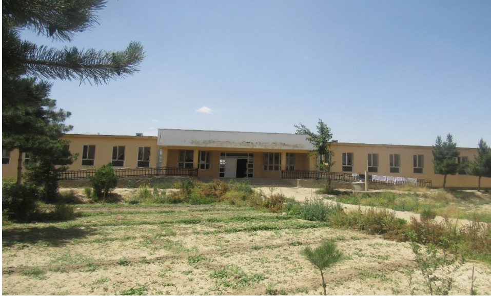
Figure 5A-59. Kabul School 30 (front view)
