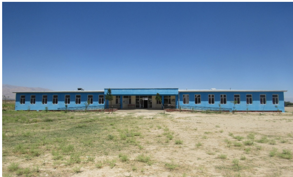
Figure 5A-61. Kabul School 31 (front view)
