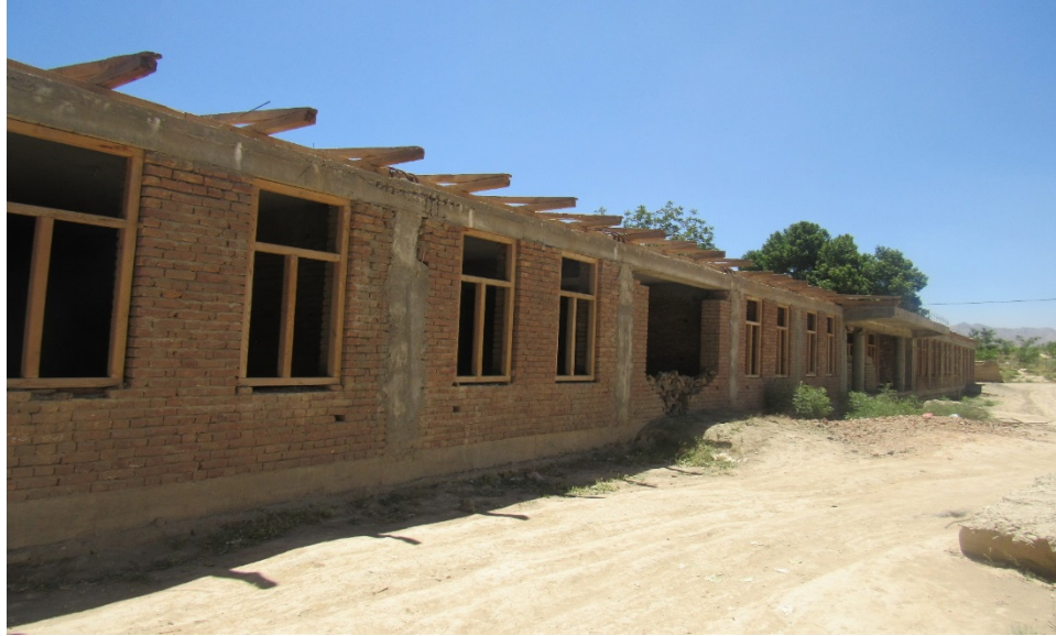
Figure A-47. Kabul School 24 (front view)
