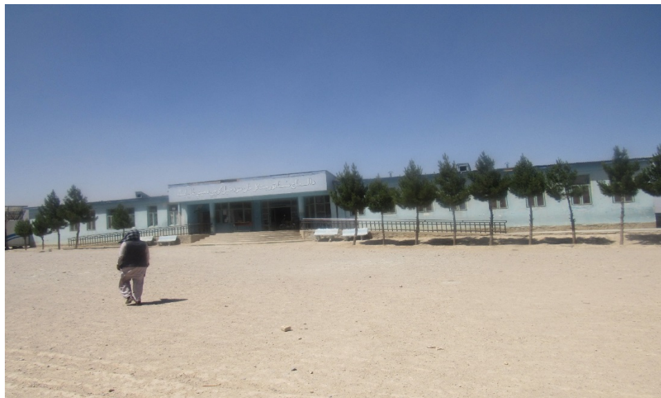
Figure 5 A-63. Kabul School 32 (front view)
