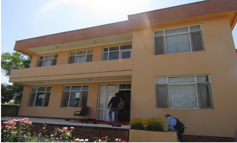
Figure A-29. Kabul School Admin 15 (front view)
