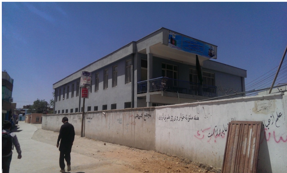
Figure 5 A-77. Kabul School 39 (front view)
