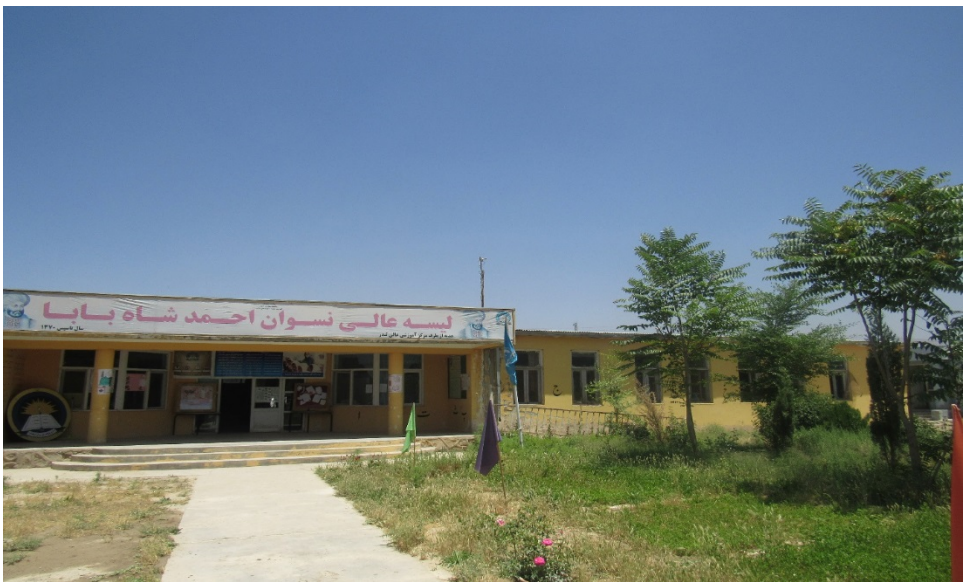
Figure 5A-69. Kabul School 35 (front view)
