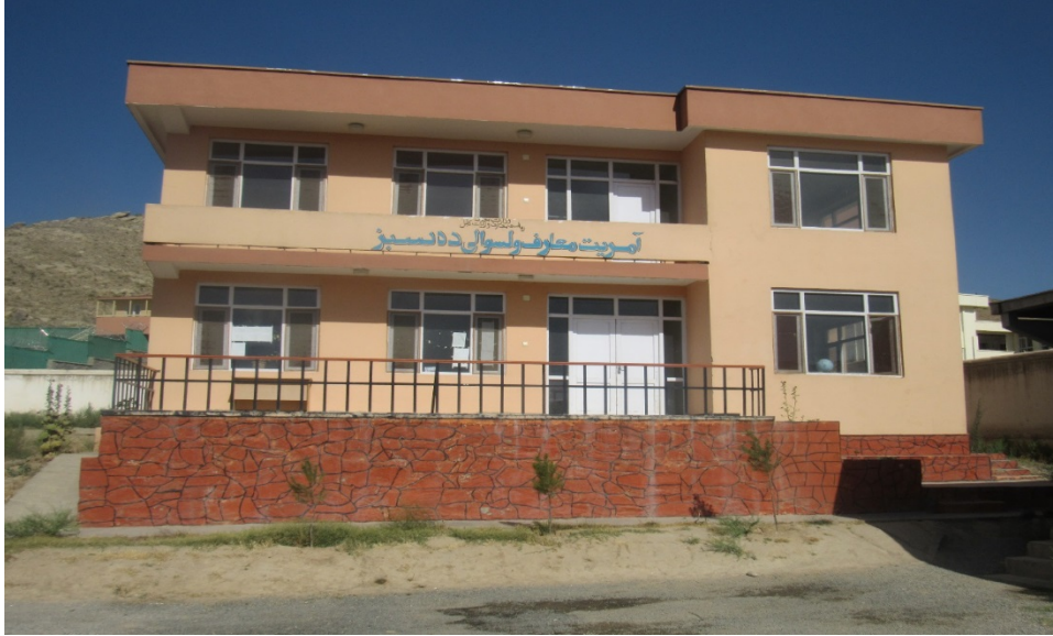
Figure A-35. Kabul School Admin 18 (front view)
