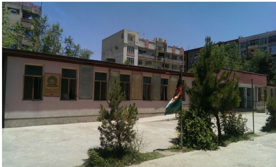
Figure A-75. Kabul School 38 (front view)
