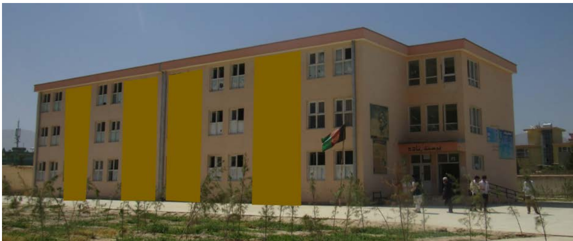
Figure C-4. Kabul School 49 (upgraded with solid masonry infill walls) (front view)
