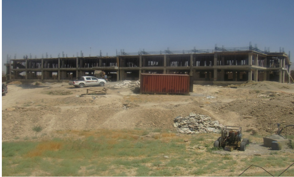
Figure A-57. Kabul School 29 (front view)
