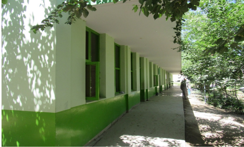
Figure A-43. Kabul School 22 (front view)
