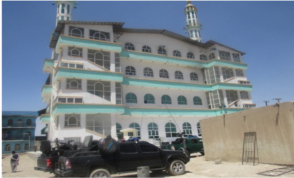
Figure A-37. Kabul School 19 (front view)
