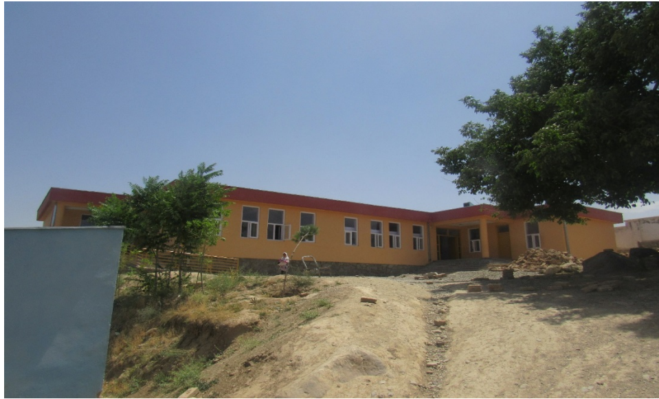
Figure A-45. Kabul School 23 (front view)
