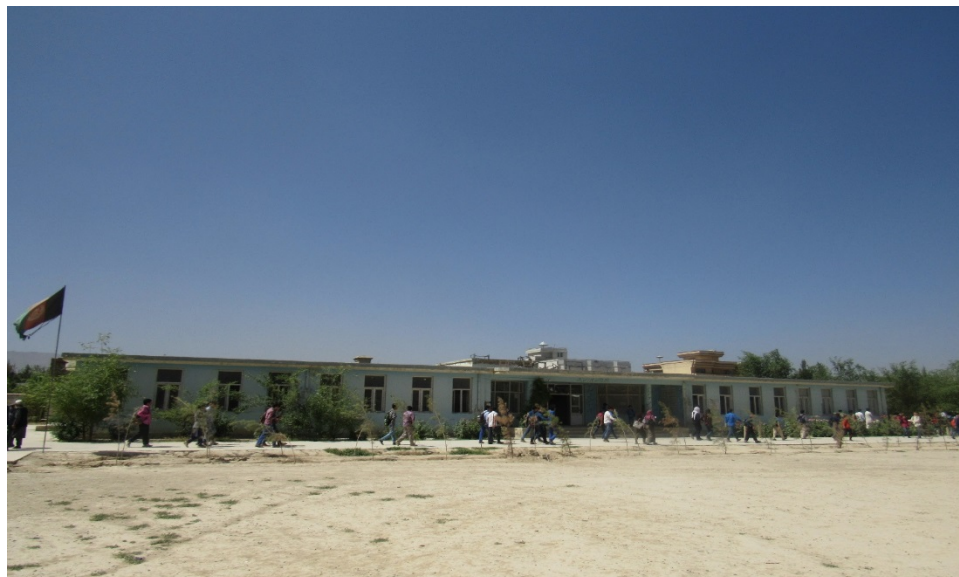
Figure 5A-73. Kabul School 37 (front view)
