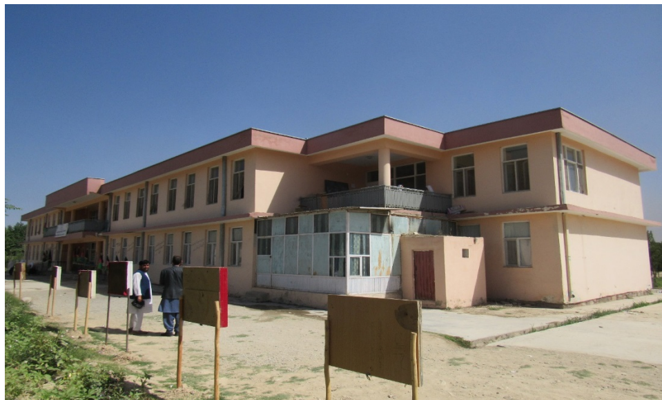
Figure A-15. Kabul School 8 (front view)
