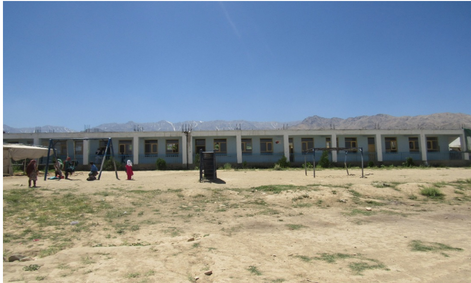
Figure A-51. Kabul School 26 (front view)
