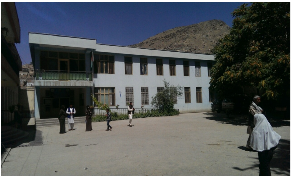
Figure A-9. Kabul School 5 (front view)
