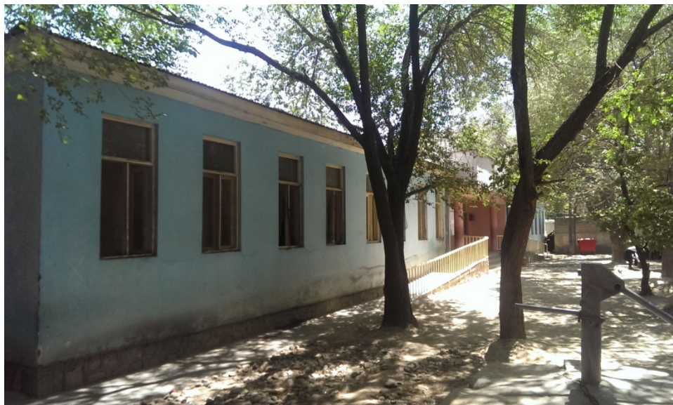
Figure A-67. Kabul School 34 (front view)
