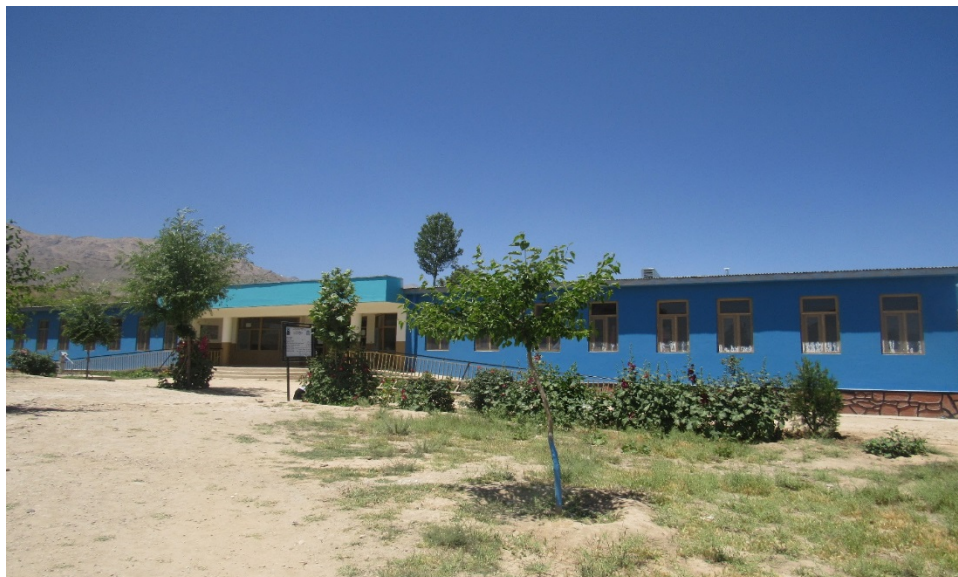
Figure A-65. Kabul School 33 (front view)
