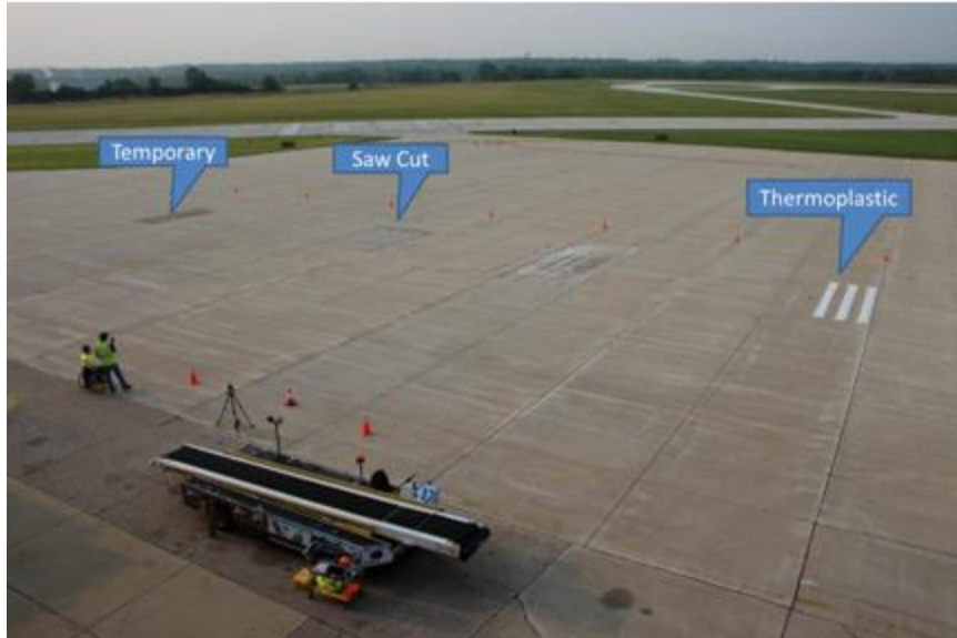
Figure 17. Rumble strip test bed from 2015 at KLAf
