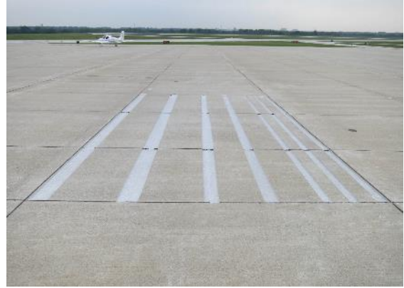
(b) Saw Cut
