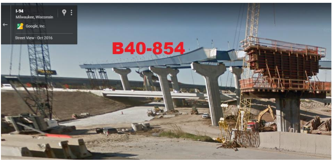
Figure 139 B40-854 under construction in October 2016
