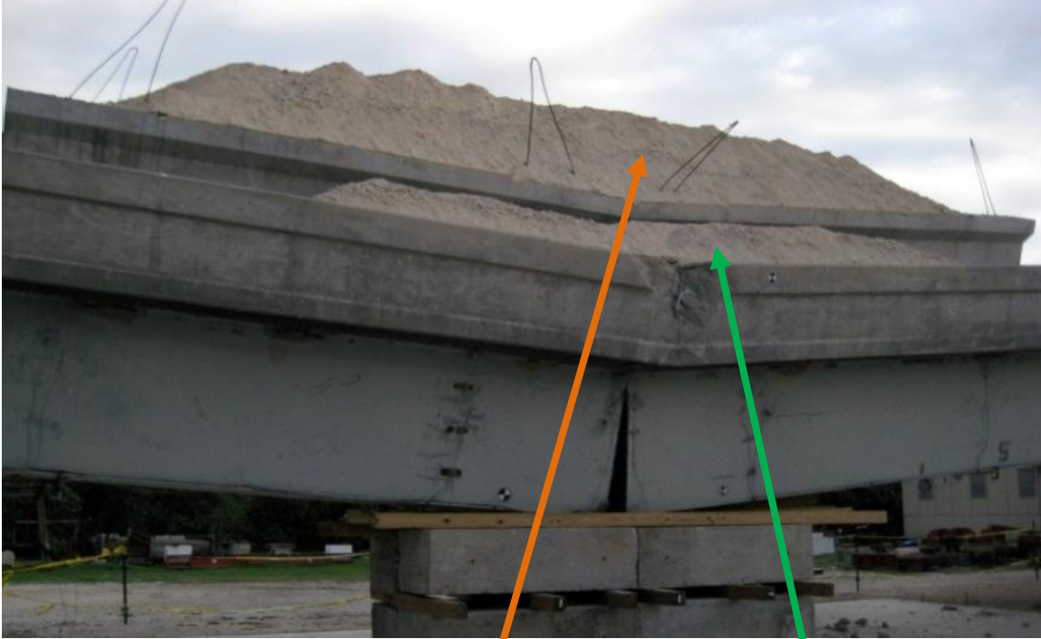
Figure 71 Test-3 details of the UT T-rib Girder Bridge from Neuman (2009) [3]
