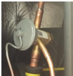
Thermal Expansion Valve
