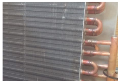
Finned-Tube Condenser
