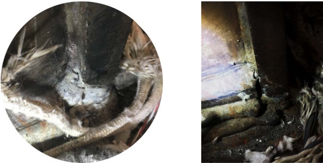
Figure 6.29 SC-W-H: Weld fracture initiated at other corners of the specimen (observed after 2\Delta_y heated cycles)
