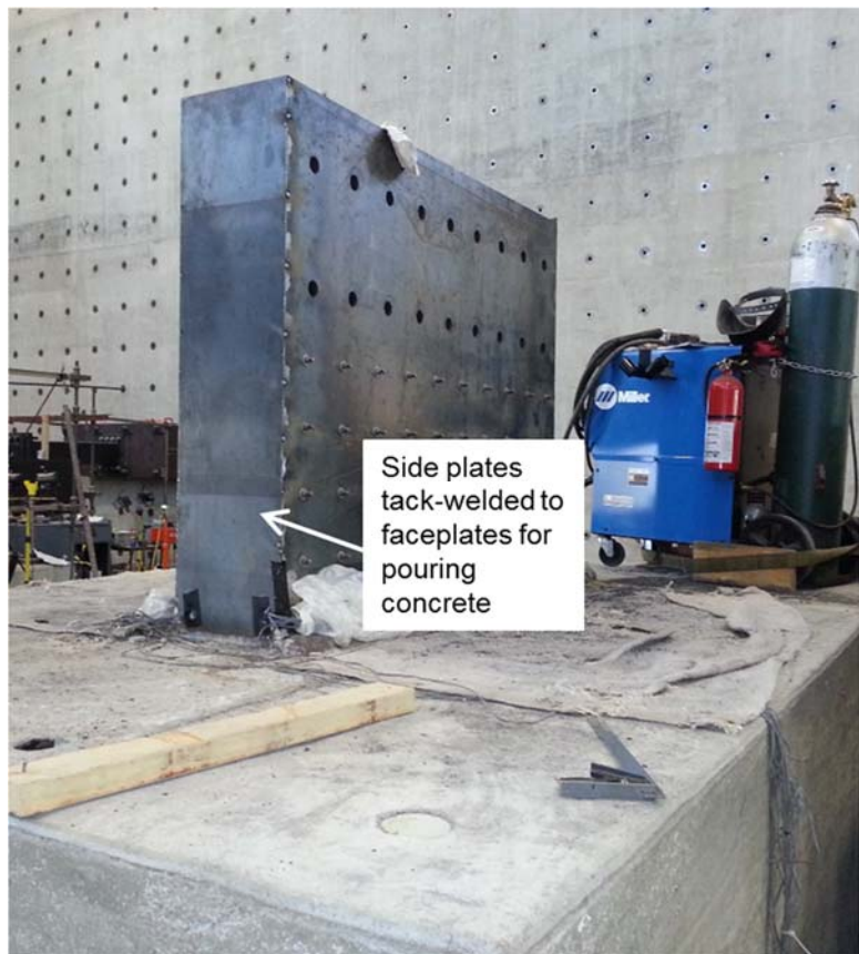
Figure 3.14 Steel assembly before pouring concrete
