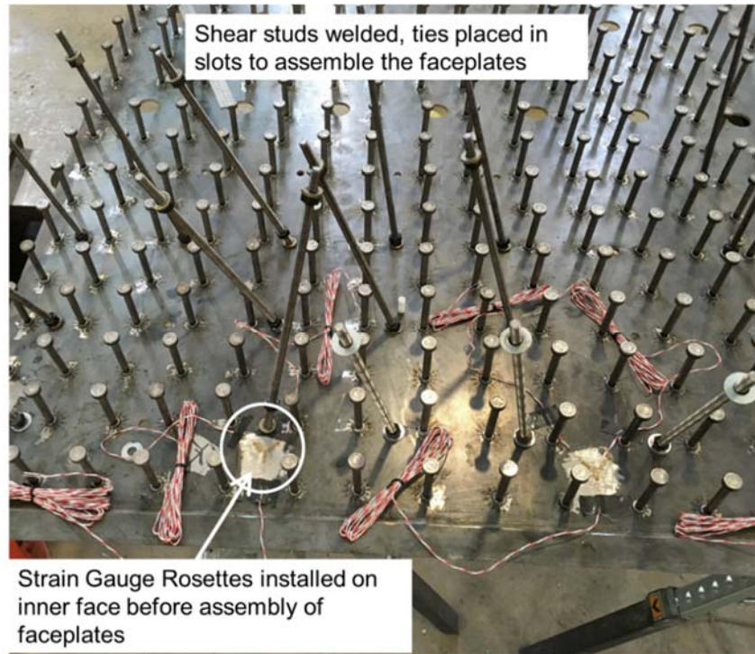
Figure 5.21 SC-WP-H: Faceplate with studs and strain gauges installed
