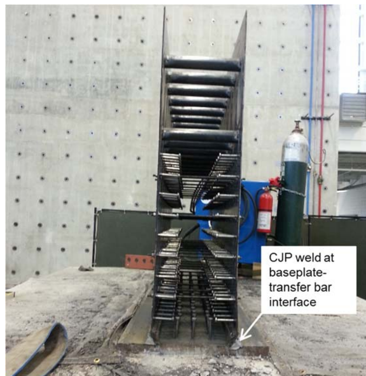
Figure 3.13 Steel assembly after welding
