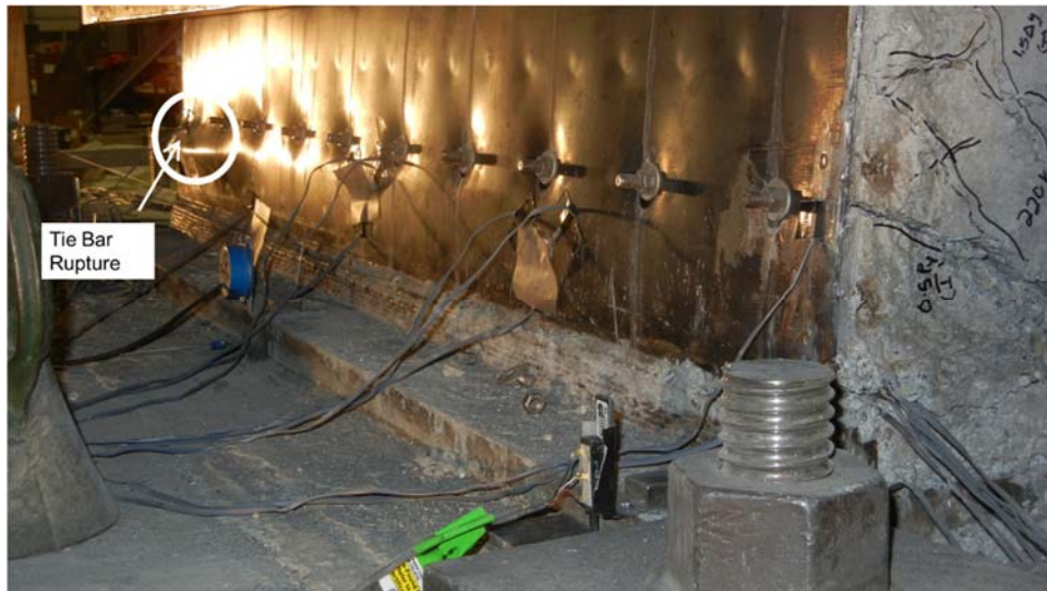
Figure 4.15 SC-0.5T-Vn: Tie bar rupture at failure
