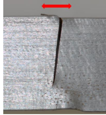
Front view of the crack.
