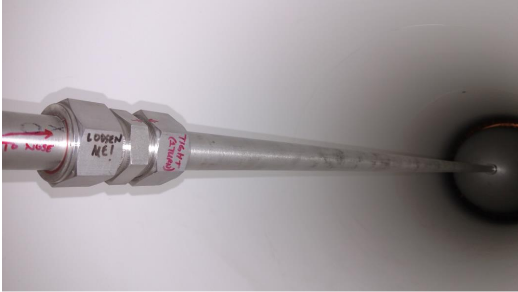
Figure 4-6. Photograph of Pipe Connecting to Nose Cone Cavity
