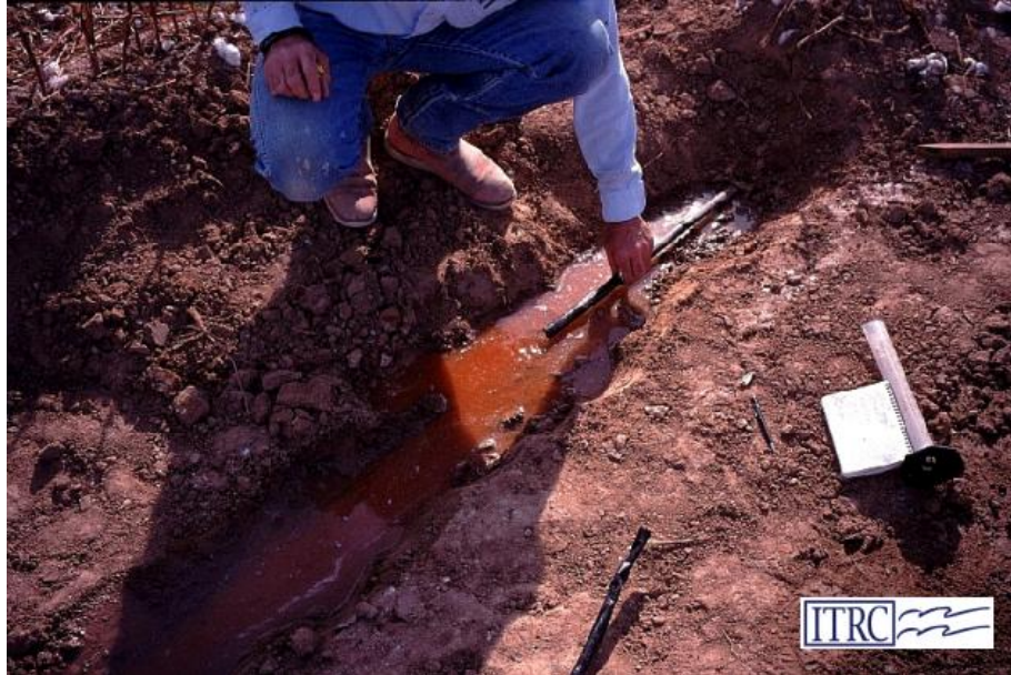
Figure 19. Chemical precipitate being flushed from drip tape. A yet-to-be-identified chemical was mistakenly injected downstream of the filters. The system plugged and needed to be replaced. This was considerably more expensive than cleaning a dirty filter.
