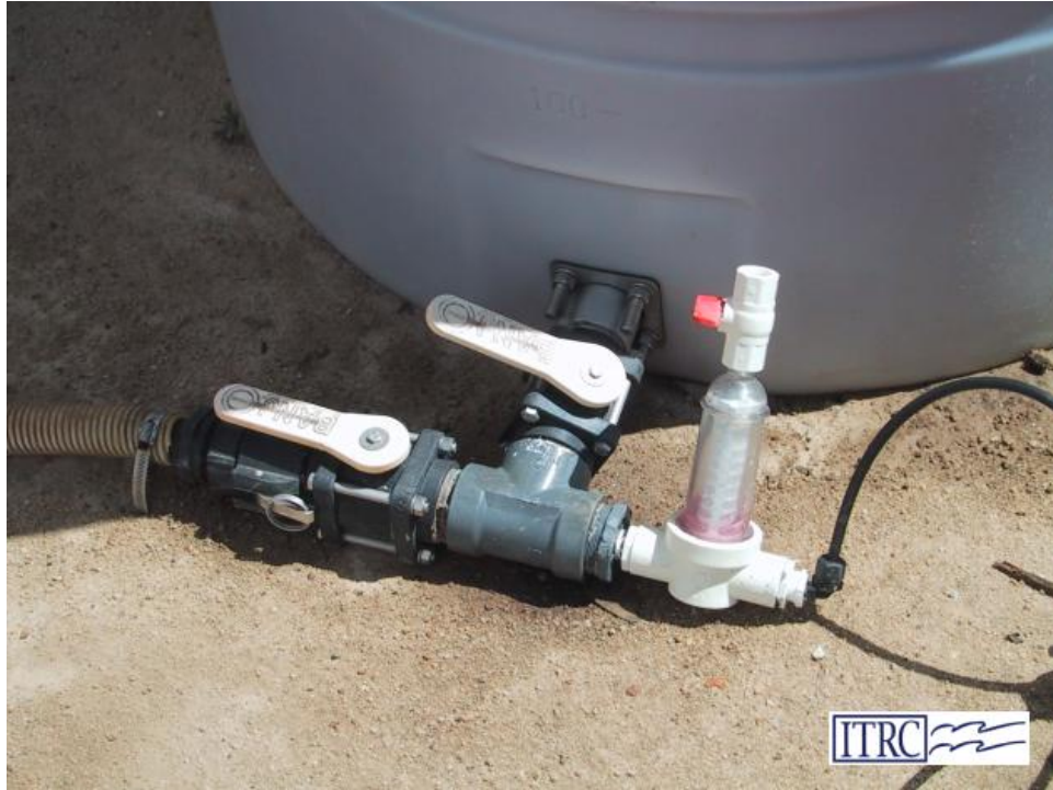
Figure 4. Recommended connection to a chemical tank. The chemical moves from the center tank through the filter and then through the chemical line to the injector pump. Fresh water can be supplied from the left hand side. The figure shows ball valves in positions that shut off the chemical and allow fresh water to flush the filter and injector.
