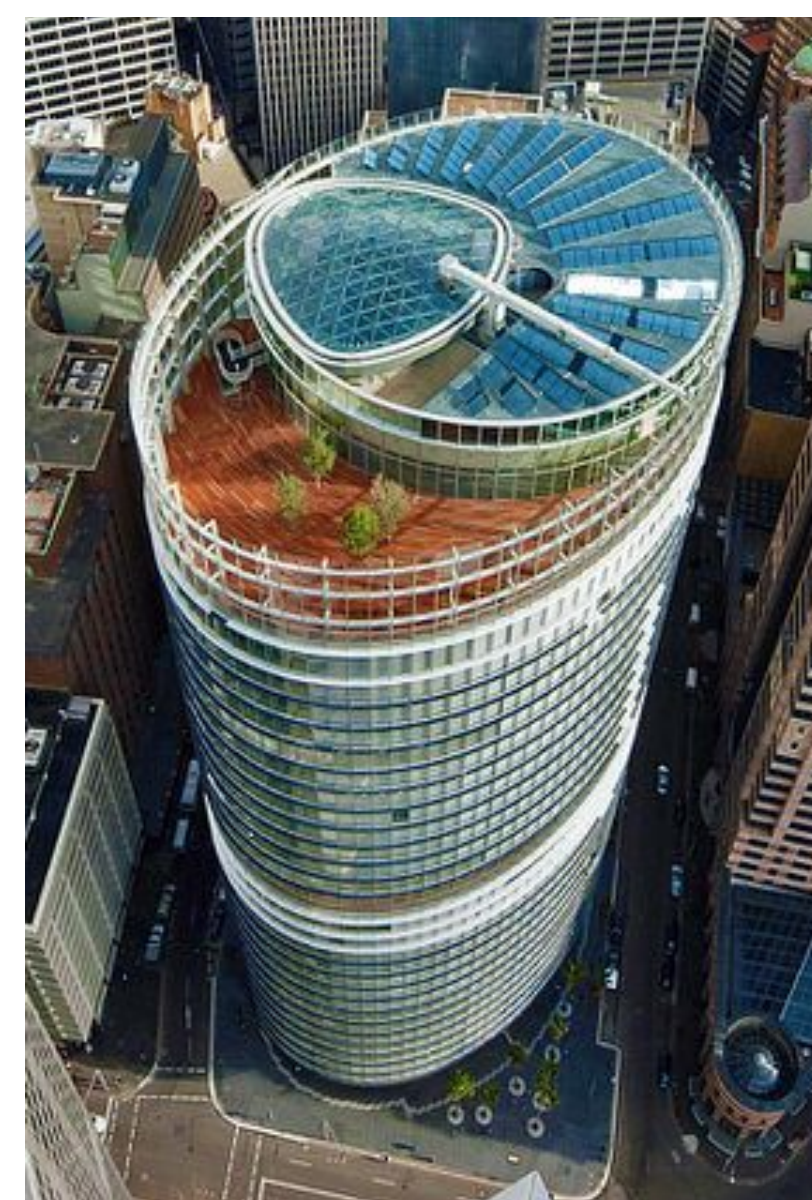
1 Bligh Street in Sydney, Australia recycles more than 100,000 liters of blackwater daily
