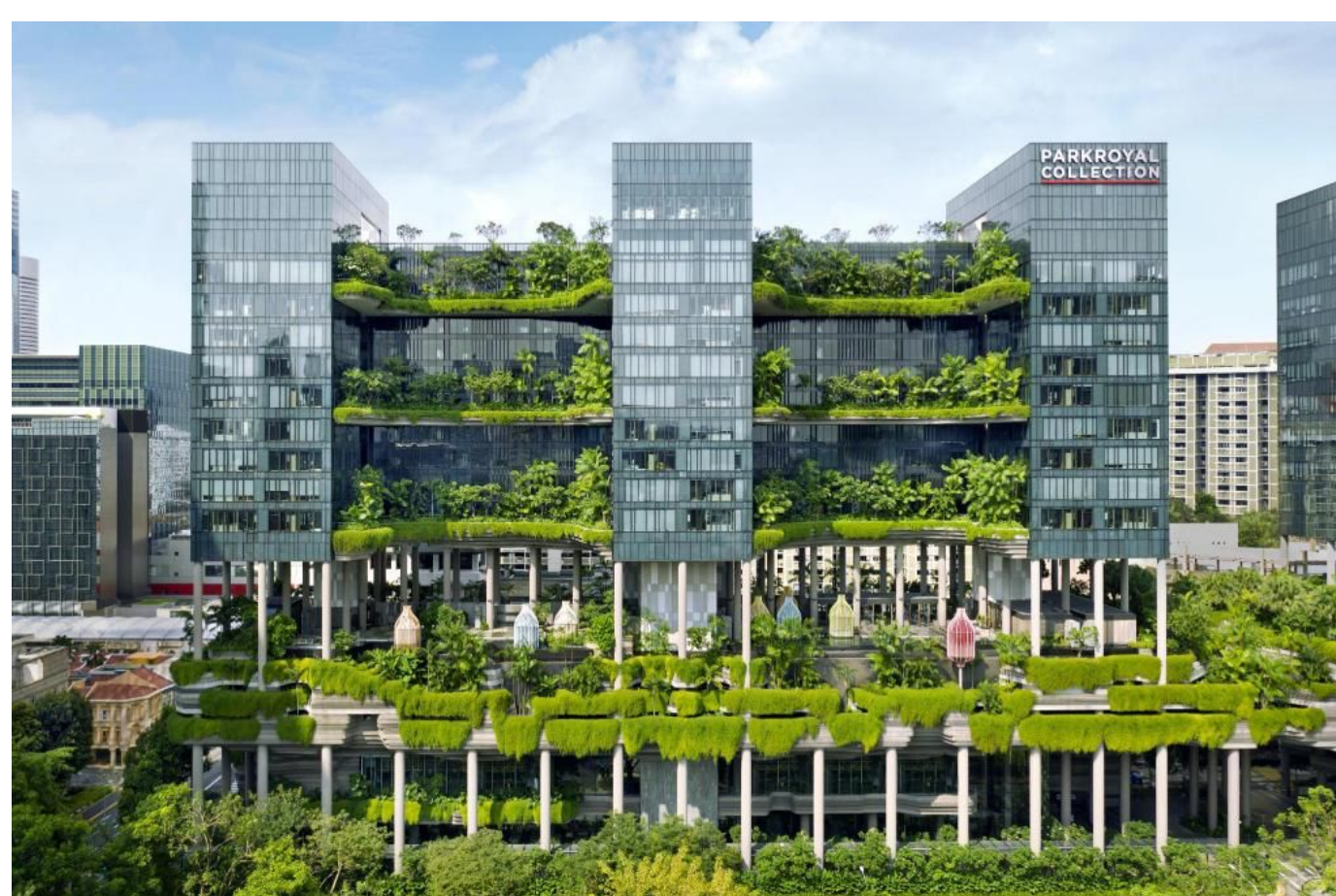
Singapore's Parkroyal Resort exterior façade and living walls
