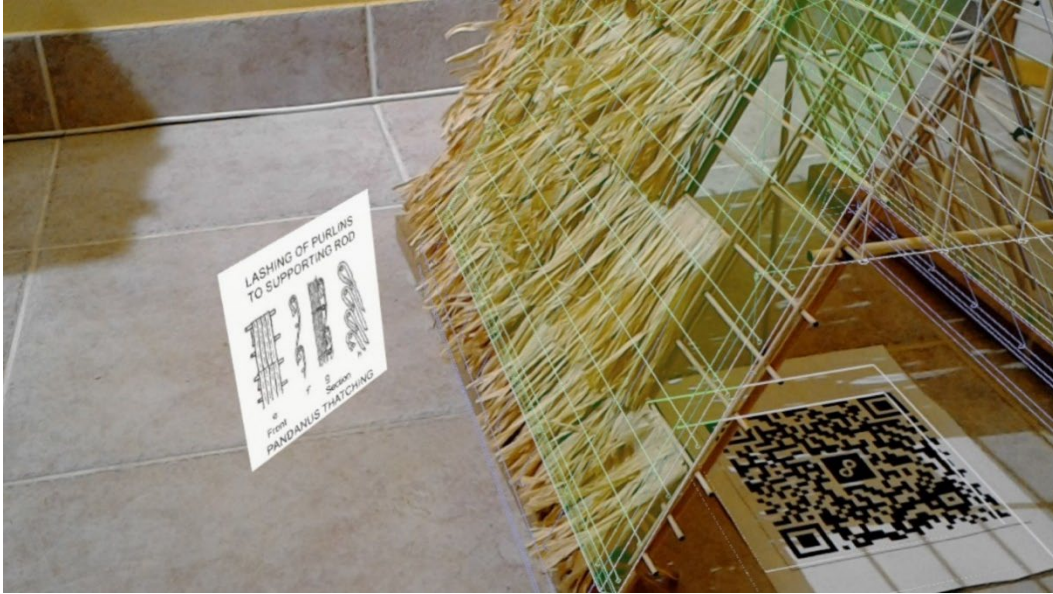
Figure 64. The Layering of the Thatching on the Purlins Following Thatching Diagram
