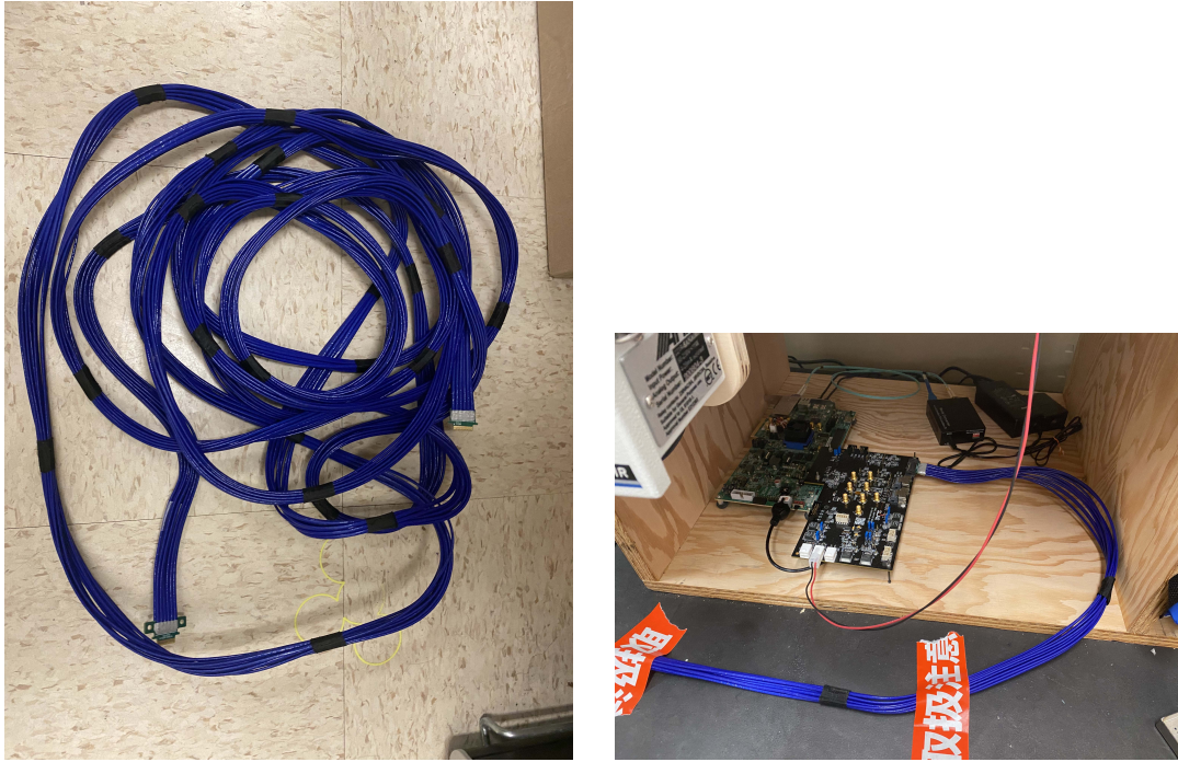
Figure 6.4 The longer cable is 11 meters, while the shorter is 3 meters long. The 3 meter cable will be used in the ICEBERG tests, while the longer cables are planned for the final DUNE FD. As communication with FEMB is currently reliant on the 3m cable, drivers will be tested to upgrade to a 11m cable in the future.
