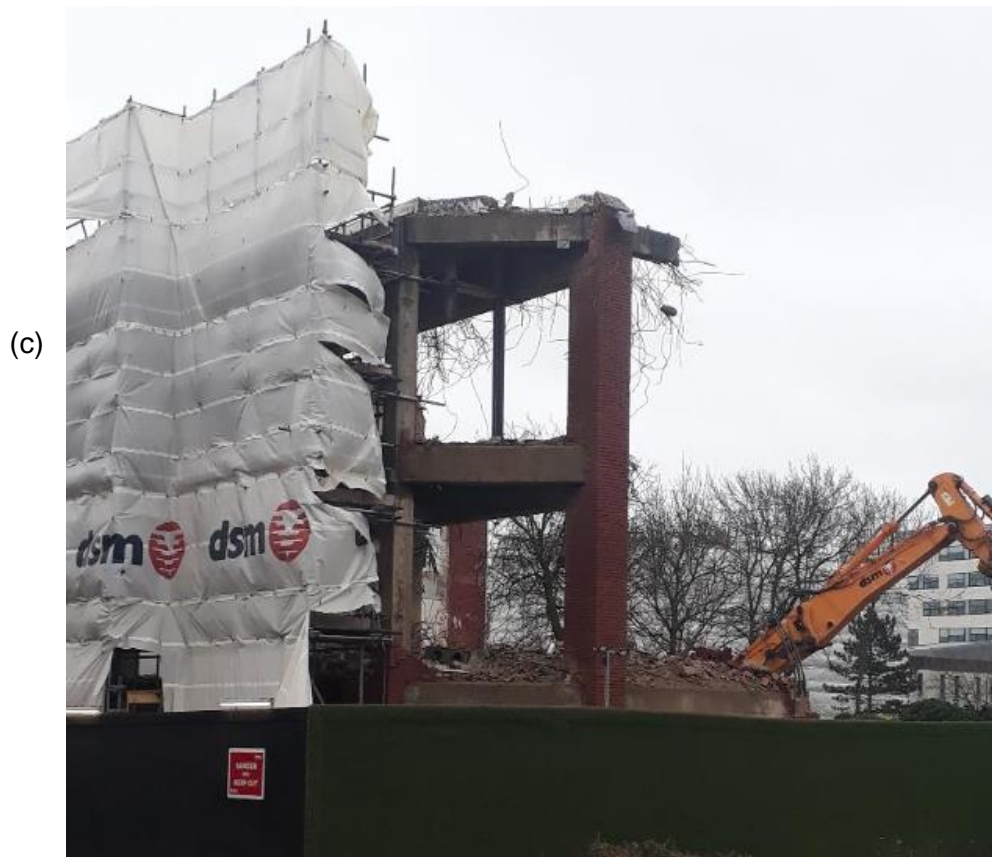
Figure 1.4: Ongoing demolition of "healthy" structures in and around Coventry University.
