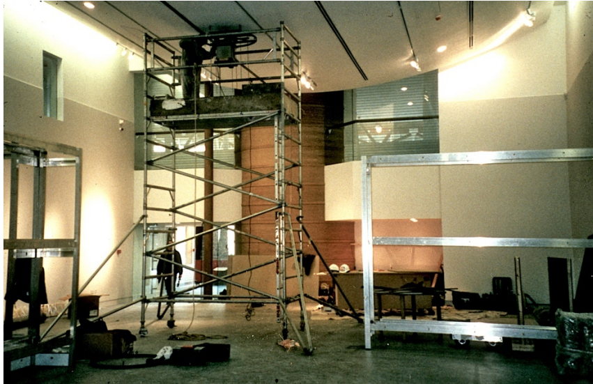
Spin, Aberystwyth Arts Centre, 2001, installation in progress. Source: Author.
