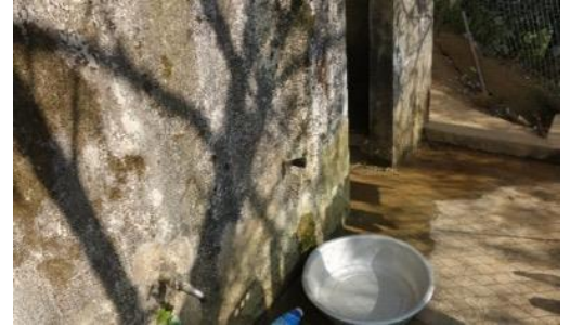
Running water pipe connected to the house.
