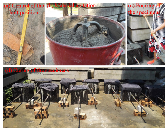
Fig. 1. Pouring and curing of pulling specimens.
