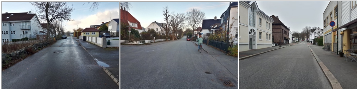
Figure 4.5 - Non-separated cyclist infrastructure at observation points 1 to 3 from left to right.
