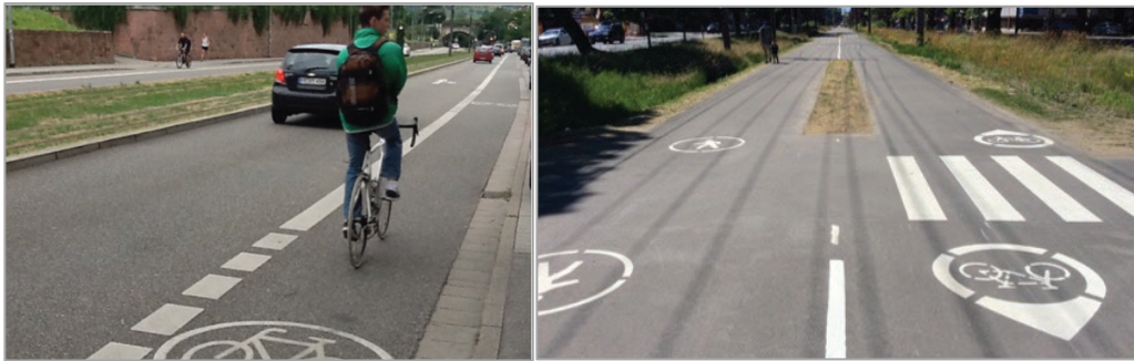
Figure 3.2 - Examples of separated infrastructure at varying degrees, bicycle lane with lane marking (visual separation) (left), bicycle path (fully separated) with designated bicycle and pedestrian travel (right), from “The Canadian Bikeway Comfort and Safety (Can-BICS) Classification System: a common naming convention for cycling infrastructure” by M.Winters, M.Zanotto, G. Butler, 2020, Health Promotion and Chronic Disease Prevention in Canada , p.290,p.291.
