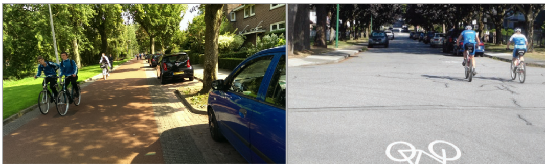
Figure 3.1 – Examples of on-road infrastructure, bicycle priority street in the Netherlands (left), from “Sykkelstrategi for Nord-Jæren 2017-2032” by R.Davidsen, I.Undheim, C.Berg, T.Dahl, R.Børresen, T.Gøtterup, pg.26, (Davidsen et al., 2016). Mixed traffic street (right), from “The Canadian Bikeway Comfort and Safety (Can-BICS) Classification System: a common naming convention for cycling infrastructure” by M.Winters, M.Zanotto, G. Butler, p.290, Health Promotion and Chronic Disease Prevention in Canada
