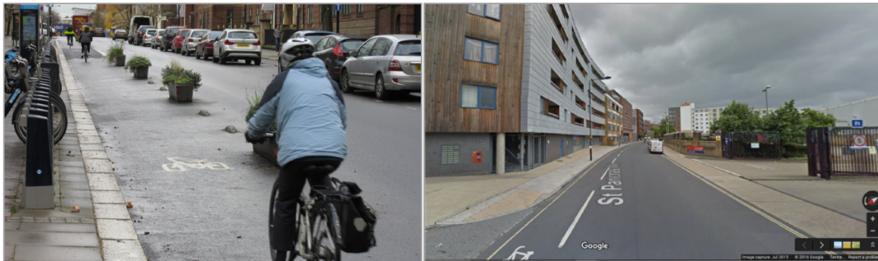
Figure 3.8 - The physically separated infrastructure (left) and the less separated control site (right), from “Diversifying and normalizing cycling in London, UK: An exploratory study on the influence of infrastructure” by R.Aldred and J.Dales, Journal of Transport & Health , 2017, p.352, p.356. Copyright Elsevier Ltd 2017.
