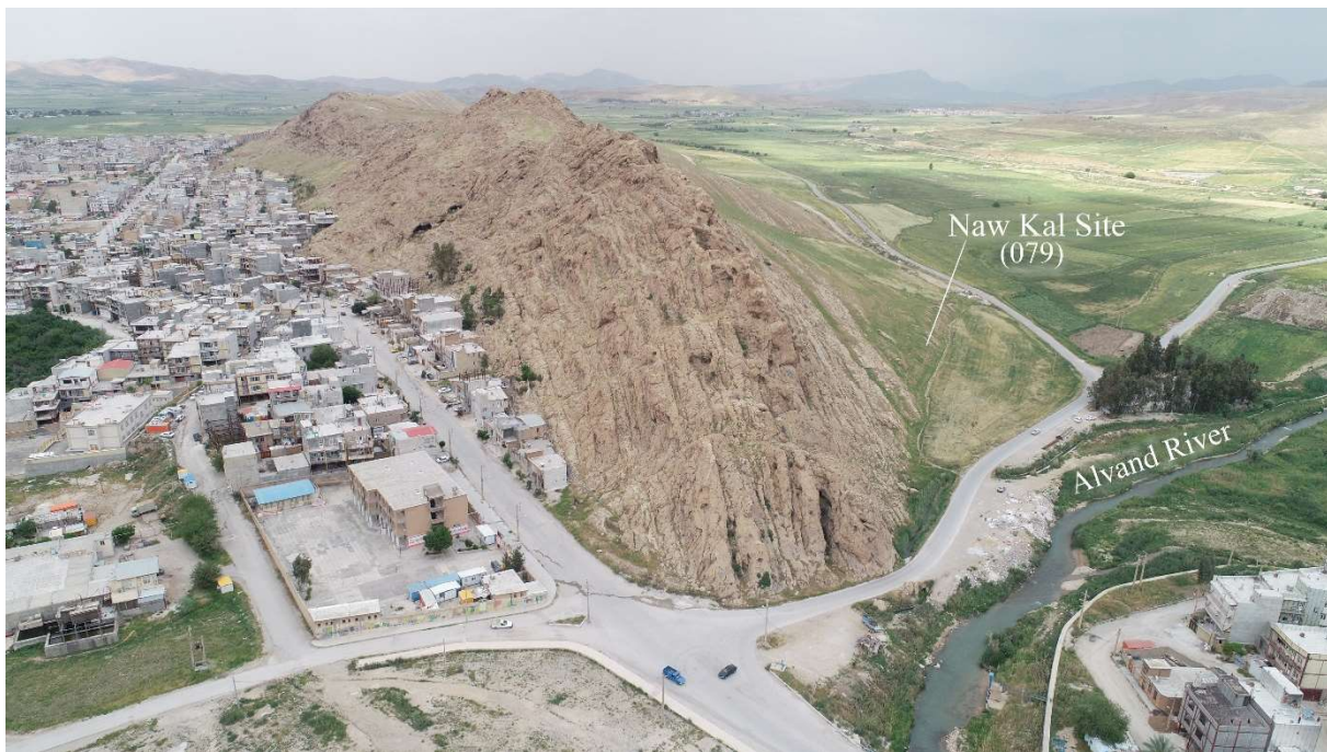
Figure 10. A view of Naw Kal showing the location of its rock mortar (courtesy of Reza Azizi).
