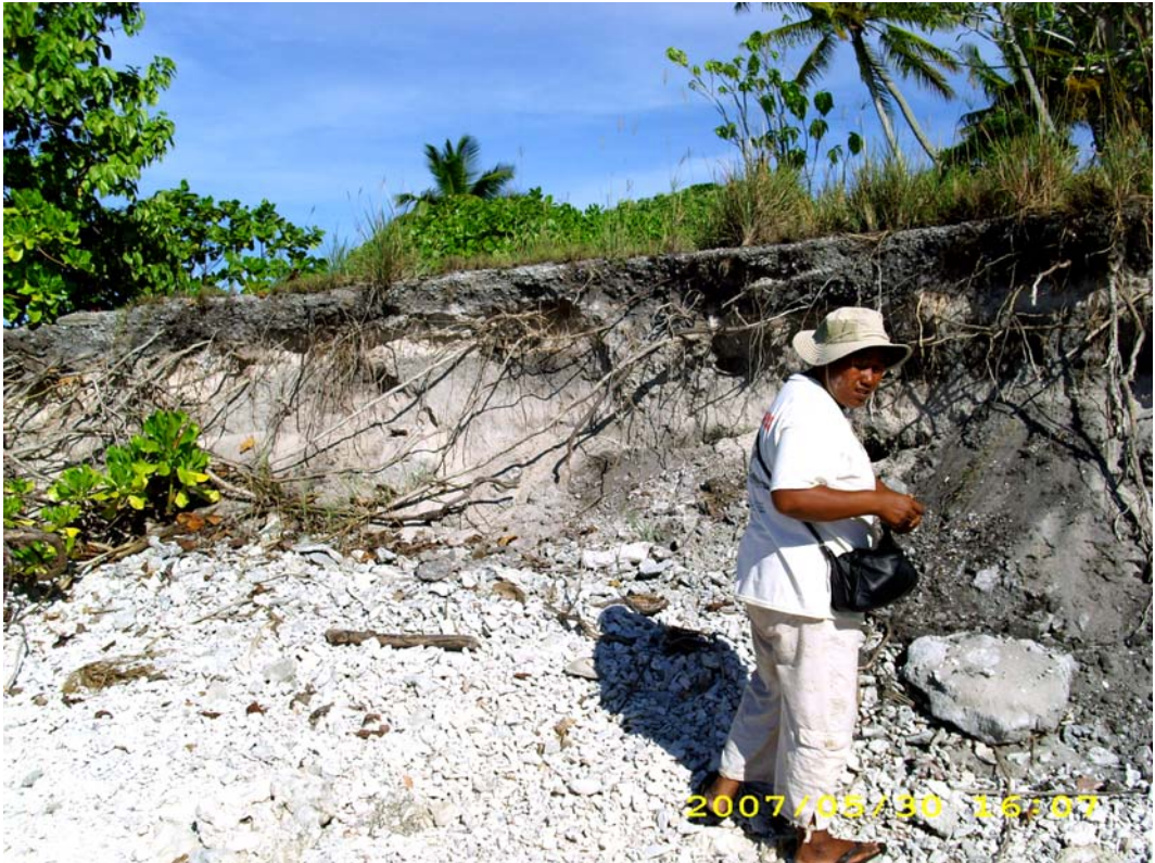
FIGURE 7. Erosional feature on Manra Islet, Abaiang Atoll.
