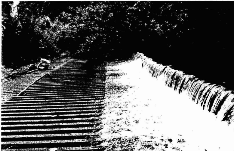
Figure 27*. Although the sugar industry is pau (ended), this diversion of 100% of Hulē'ia Stream's base flow continues to send water out of the watershed to Waita Reservoir. The streambed continues dry for a hundred yards, and then the groundwater begins to recharge the streamflow. (Photo by Adam Asquith)
