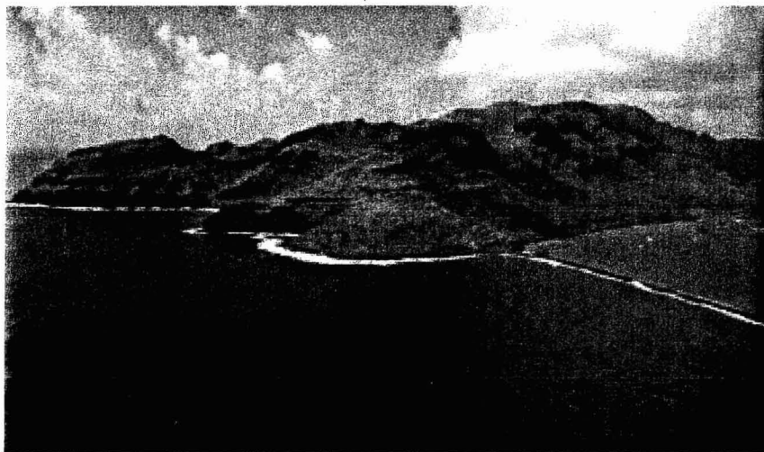
Figure 2*. The construction of the harbor at Nawiliwili has interrupted the flow of sediment out to sea, thus sediment is deposited in the harbor and on the reefs. When large surf arrives, this sediment is reintroduced into the water. Notice the difference in the color of the ocean and harbor water. Without the breakwater, the sediment would move out into the long shore flow. (Photo by David Boynton, Casey Riemer pilot - Jack Harter Helicopters. )
