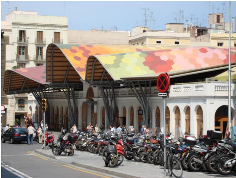
Figure 31: Barcelona, Mercat Santa Caterina exterior. With its distinctive undulating roof, the market features many of the same culinary sights and smells as the larger and better known Mercat de Sant Josep de la Boqueria. Motorcycles and bicycles parked outside serve as reminders of an emphasis on alternative transportation in Spain's larger cities. Photo: Stieve personal collection.
