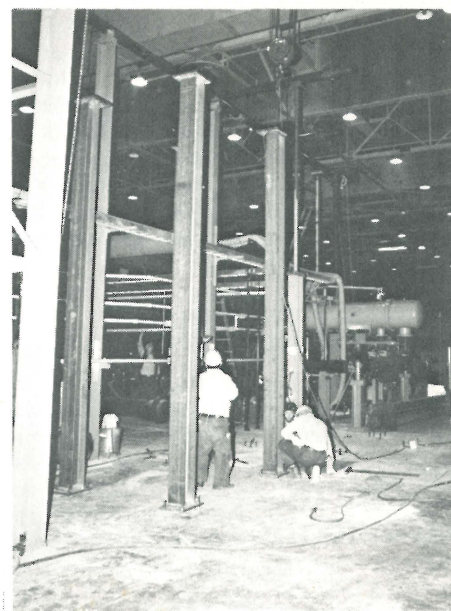
Engineers install girders which will support other heat exchangers.
