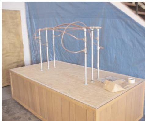
Once the base was completed, the armature was constructed on it.
