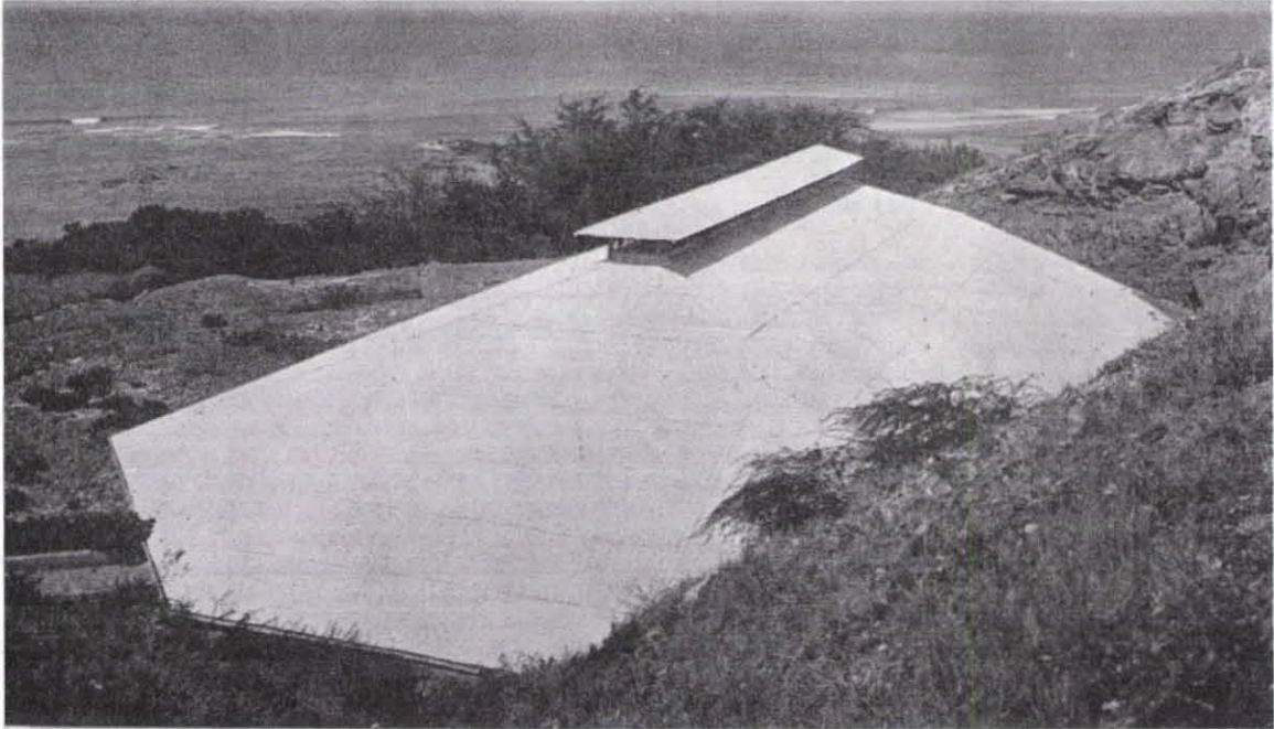
Figure 44: Diamond Head Reservoir, 1913
