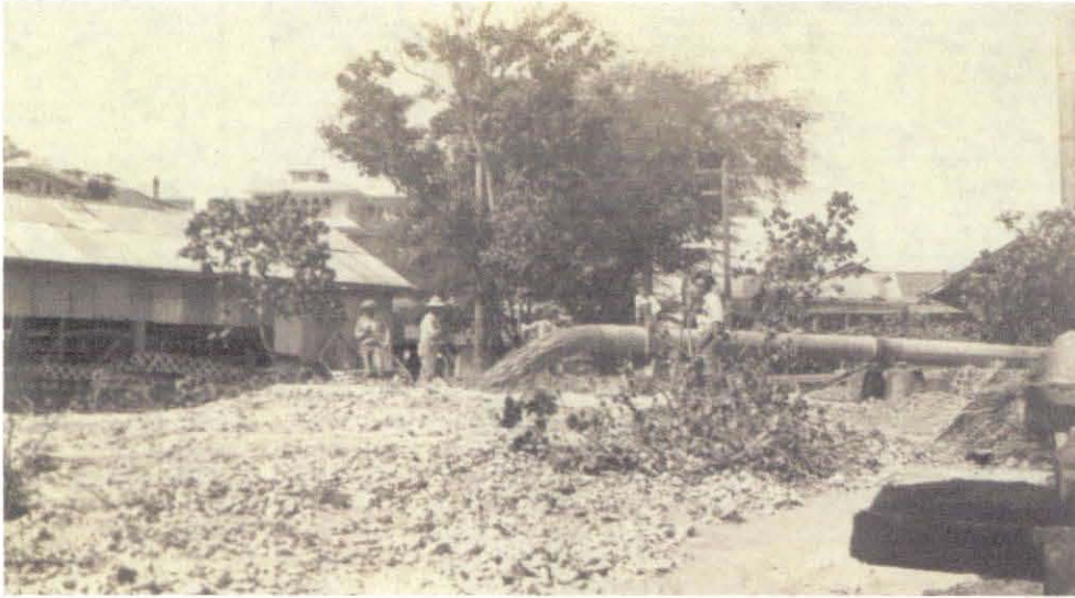
Figure 13: Fill from Ala Wai Canal dredging being used to fill in 'Āpuakēhau Stream near Moana Hotel, circa 1924
