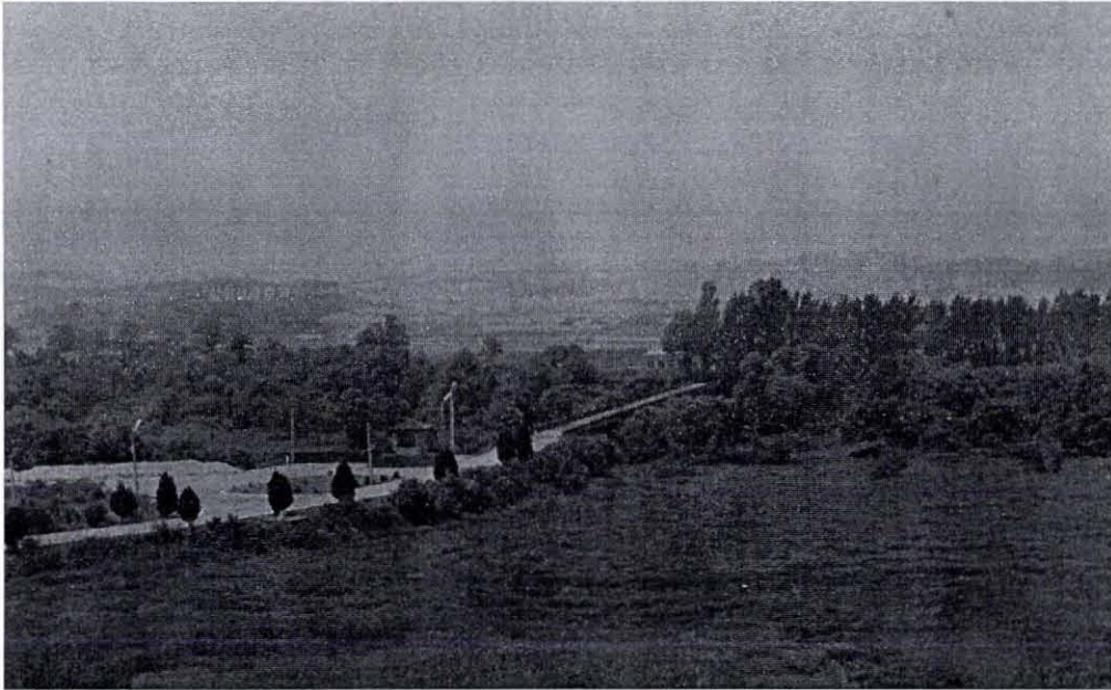
Figure 2-2. The Bridge of No Return (Source: Author's photograph)
