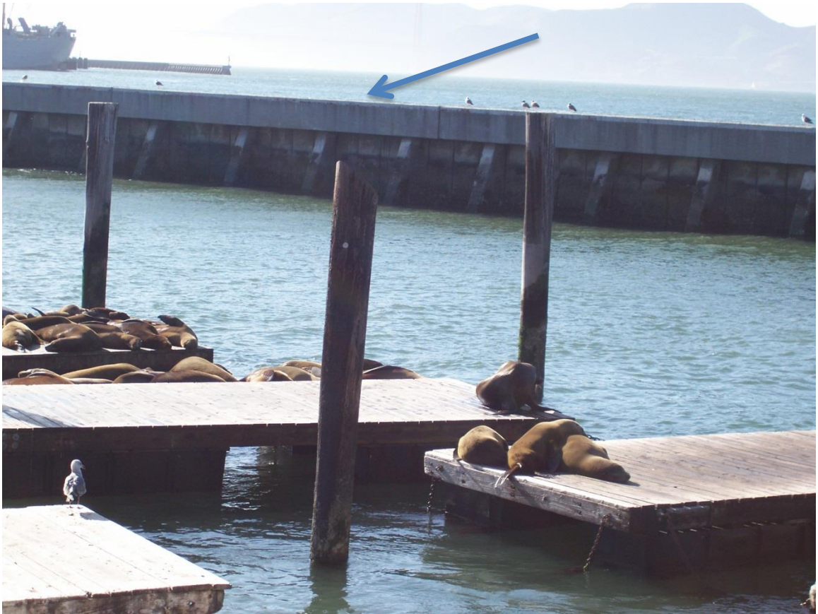
Figure 27: Sea wall that inhibits predator entrance at Pier 39
