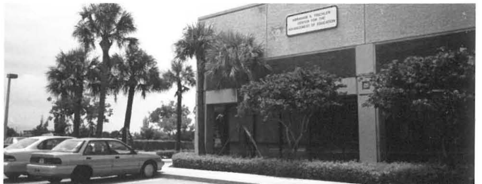
The Westport Building, located on Davie Road, near I-595, became the off-campus home of PHE and other programs of the Fischler Center for the Advancement of Education in 1991.
