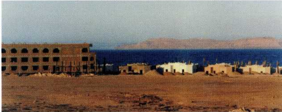
One of the first hotels under construction at Nabq Tourism Center
